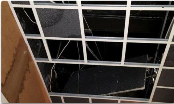
On the ceiling in the kitchen
