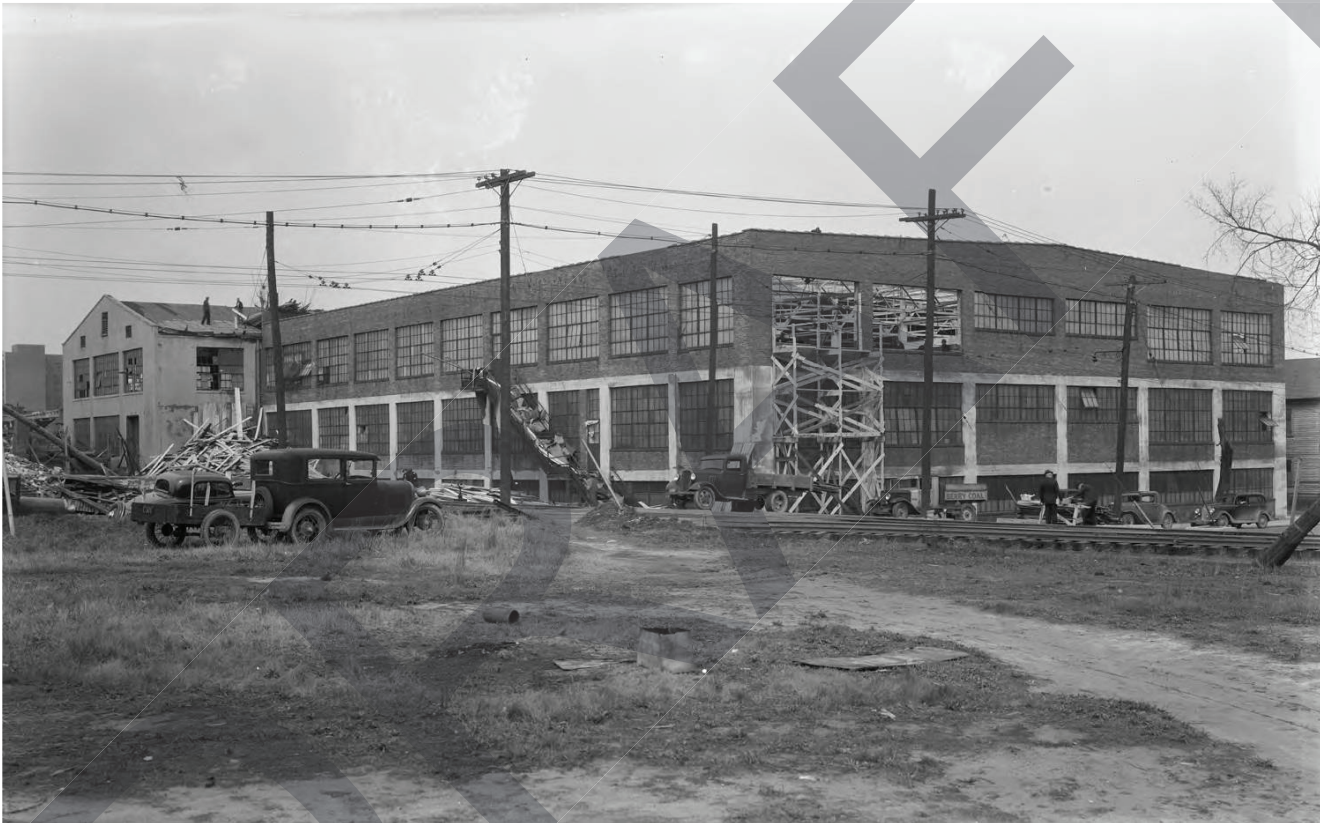
Figure 5. Construction view of Blue Bell Company Plant, south wing. Note relationship to rail tracks. Photo shows repairs being made after 1936 tornado.
