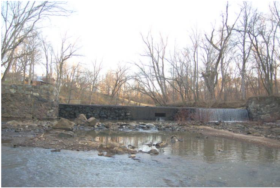
Dam, Great Alamance Creek
