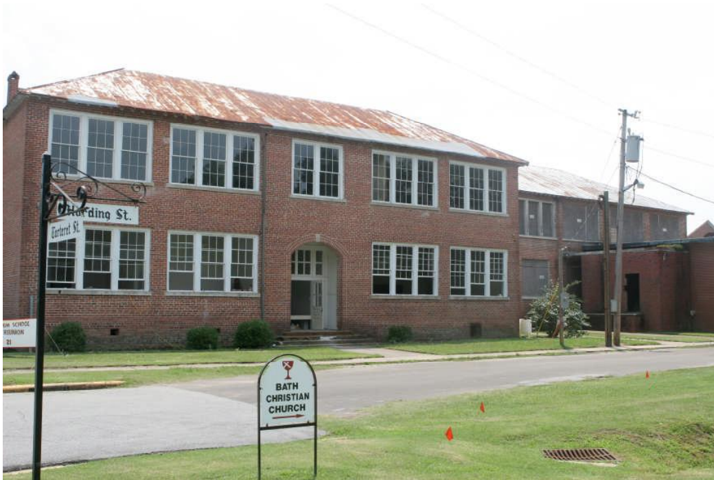
Façade view of 1920 building on left; 1918 building on right
