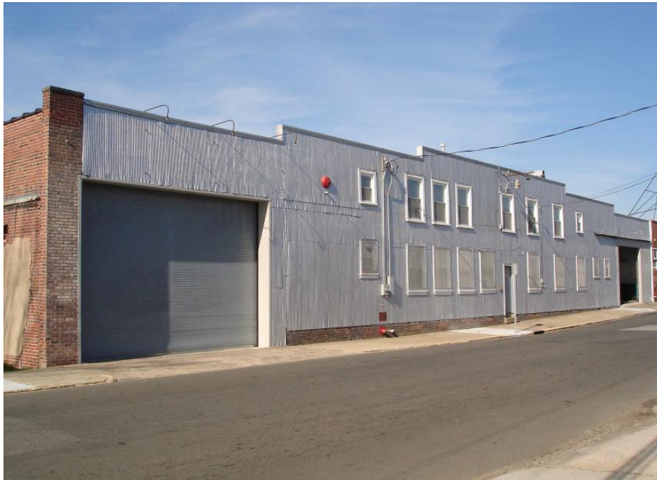
South end of facade
