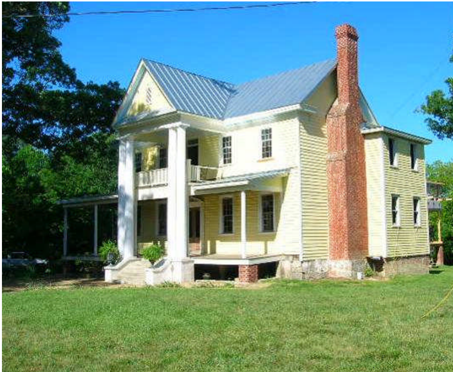
Front and side view, during rehabilitation
