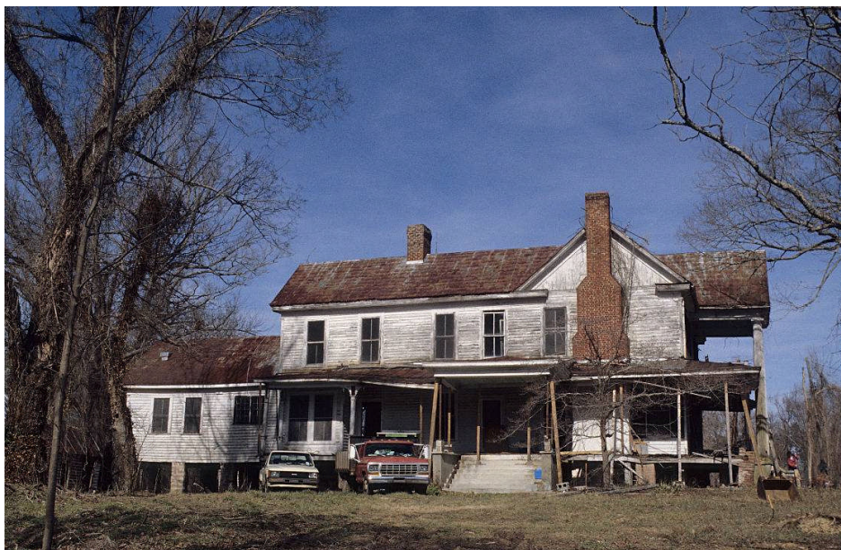
Side view, before rehabilitation
