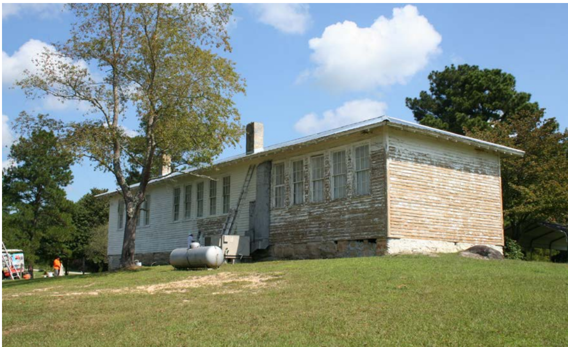
Oblique view of south and west elevations, facing northeast
