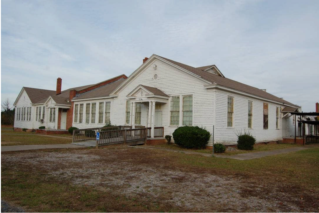
Overall view of 1941 school building
