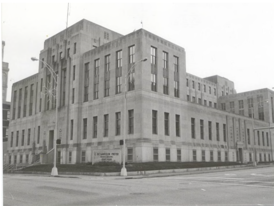
Overall rear view from West Friendly Street
