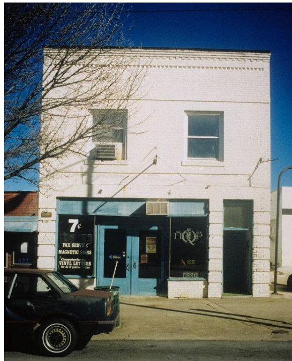
620 North Main Street, Boundary Increase Area A
