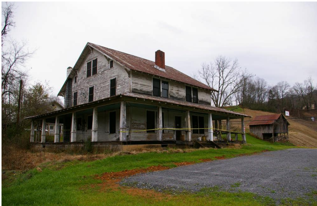
Overall front view
