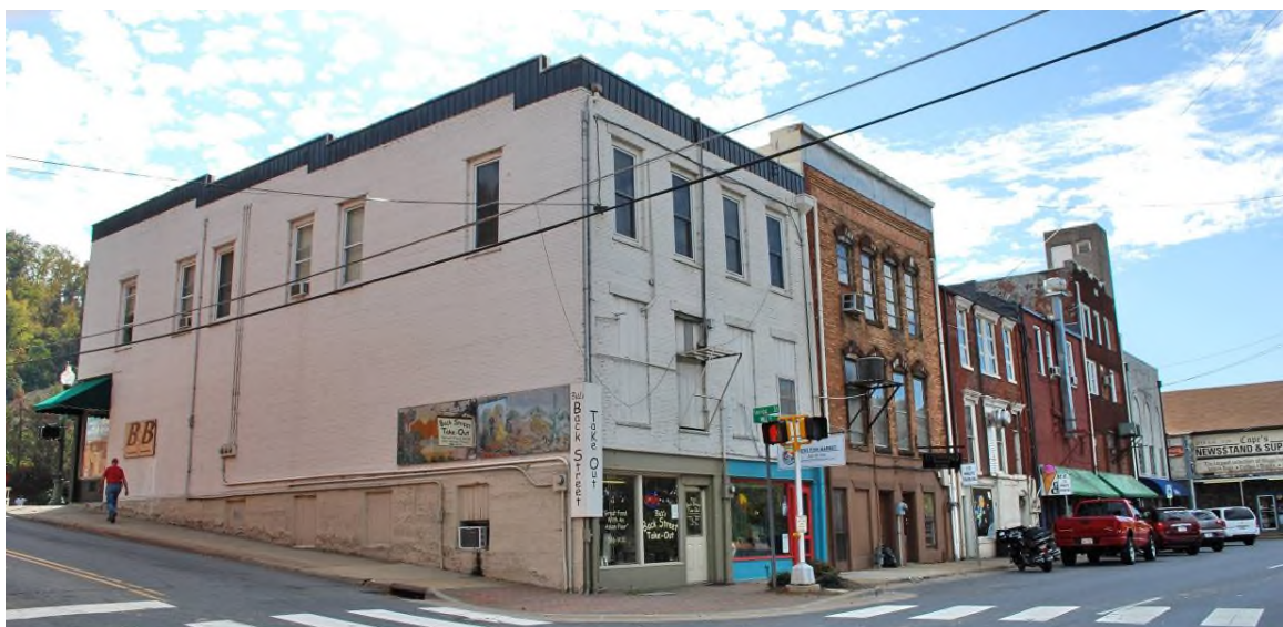
594-642 Block of Mill Street, looking west
