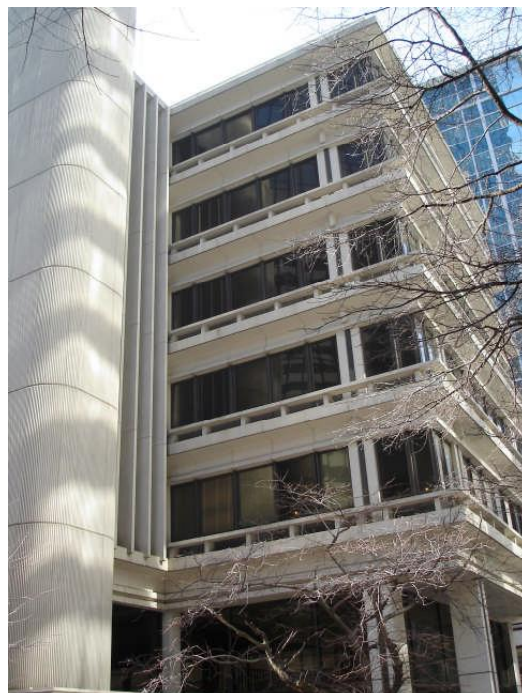
Side view with elevator tower
