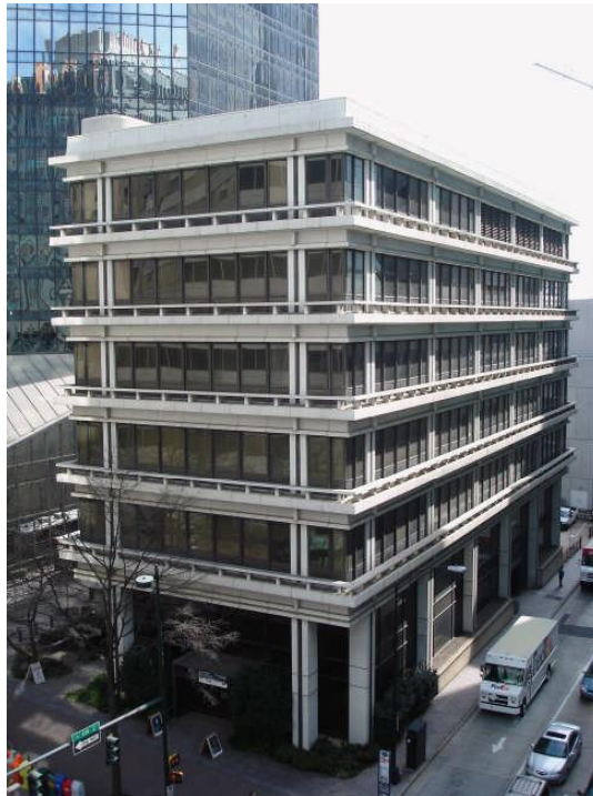
Façade and side view
