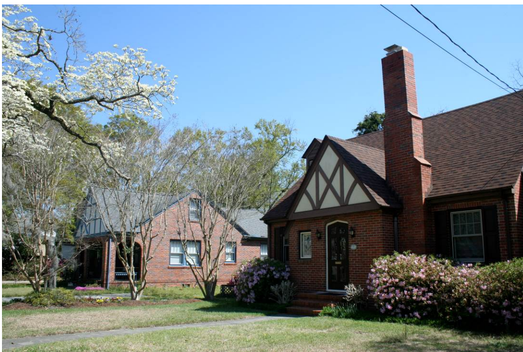
11-13 Keaton Avenue, looking northeast
