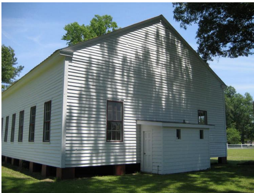
Side and rear view
