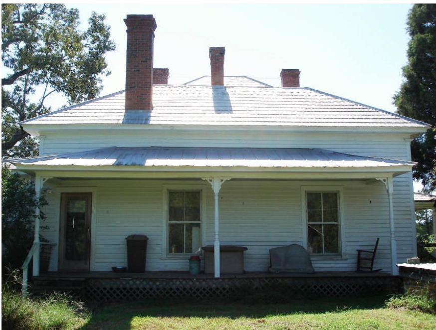
Rear view of kitchen wing
