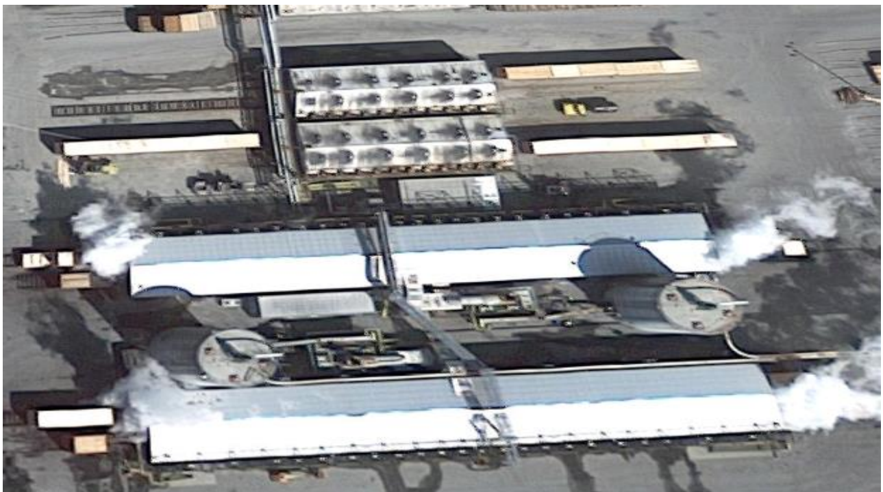
Google Satellite 3D image of the two steam-heated batch kilns (top middle), two continuous direct-fired kilns, and two fuel silos.
