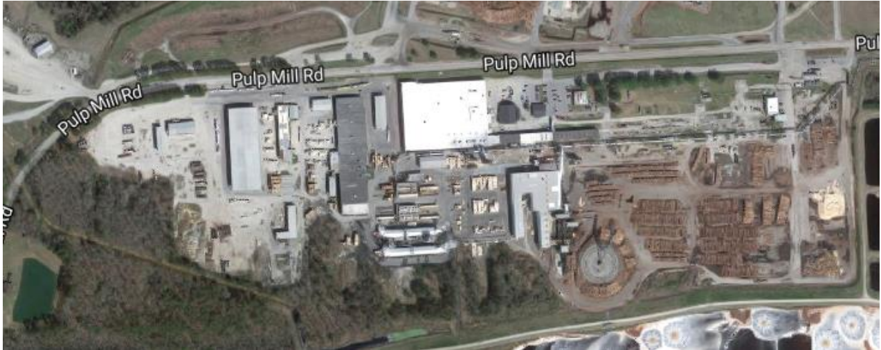
Google Satellite image of Weyerhaeuser Plymouth Lumber Mill.
