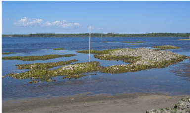
Loose oyster shell sills during construction
