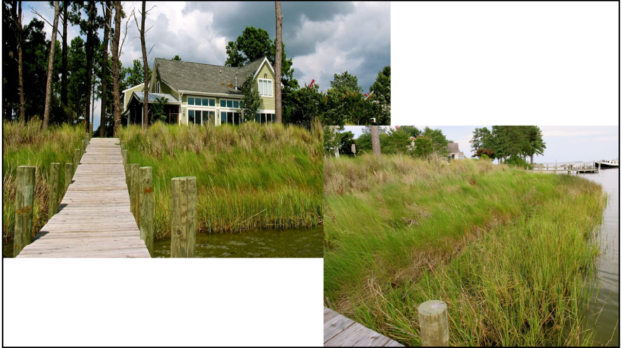
After ~18 mos, the biologs remain in place, and the banks planted with native marsh and other coastal plants have become well established, providing excellent erosion control and maintaining the benefits of a natural shoreline.
