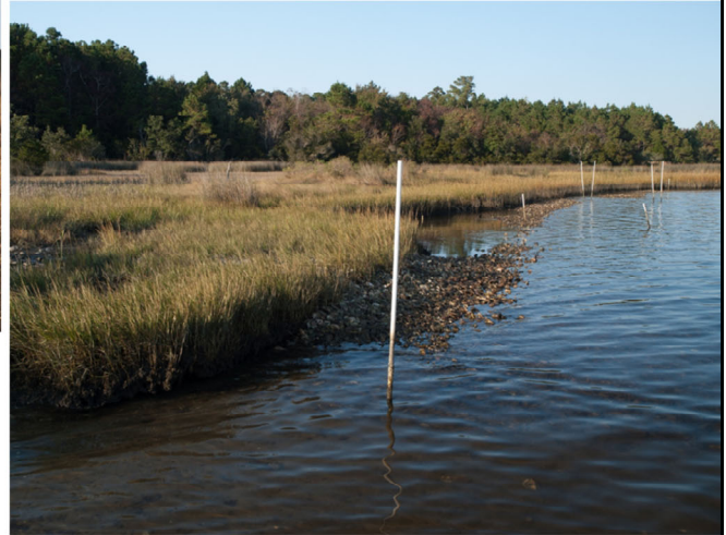
Loose oyster shell sill after Hurricane Matthew
