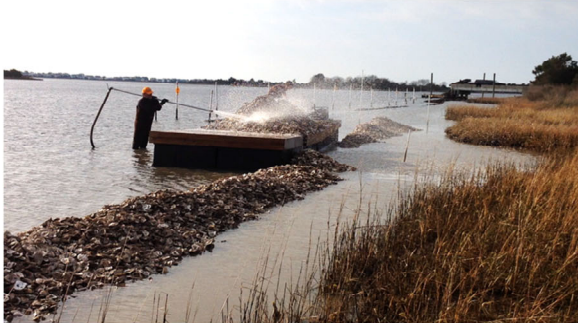
Loose oyster shell sills during construction
