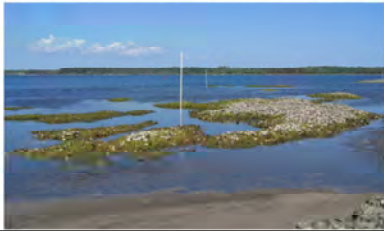
Loose oyster shell sills during construction
