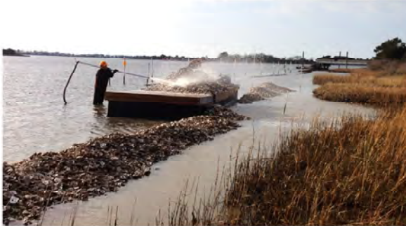
Loose oyster shell sills during construction
