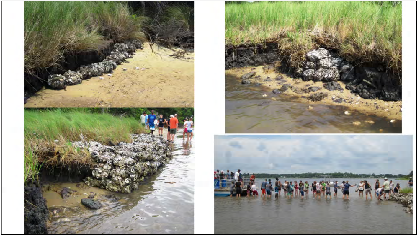
This marsh toe revetment, constructed from bags of loose oyster shell, was built by volunteers.
