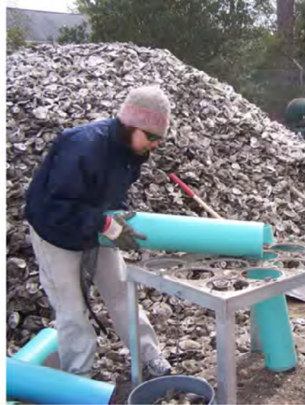
Step 2: Pull bags over PVC tubes
