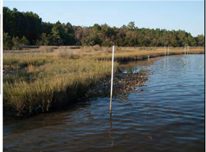
Loose oyster shell sill after Hurricane Matthew
