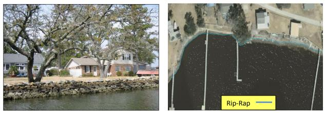
Figure 11: Examples of rock revetments.
