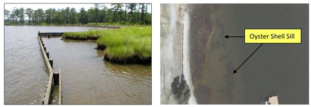
Figure 10: Timber sill protecting an existing marsh (left) and oyster shell sill from aerial photo (right).
