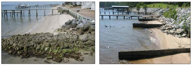
Figure 8: Rock groin covered in oyster shell (left) and series of timber groins (right).
