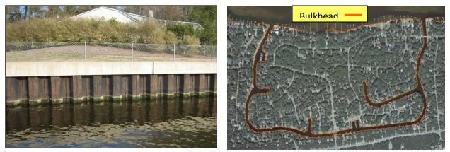
Figure 12: Steel sheetpile bulkhead (left) and digitized bulkhead from aerial photo (right).
