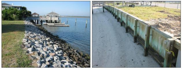
Figure 5. Modified shoreline with a riprap revetment (left) and wooden bulkhead (right).
