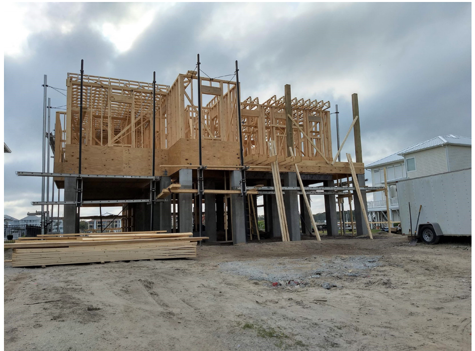
Although no building code regulations can completely protect against rising seas and increasingly damaging storms, significant elevation of new structures will help reduce vulnerability to stormwater flooding.
