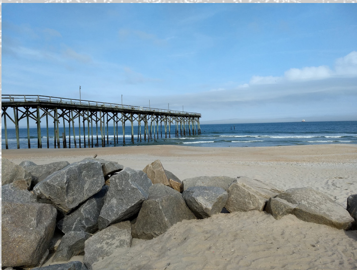
The pier on the North End.
