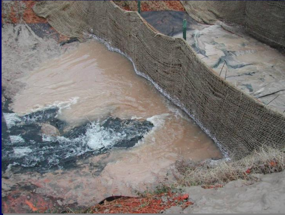
PAM sprinkled on coir baffle in basin (maybe)
