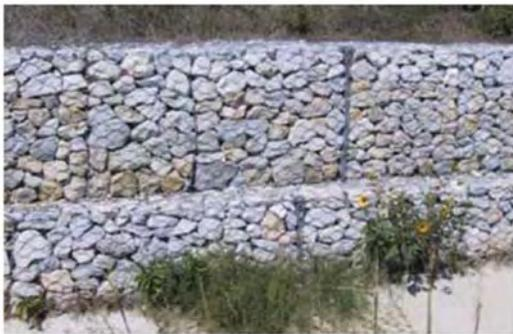
**Figure 6.73e** Vegetated gabions under construction
