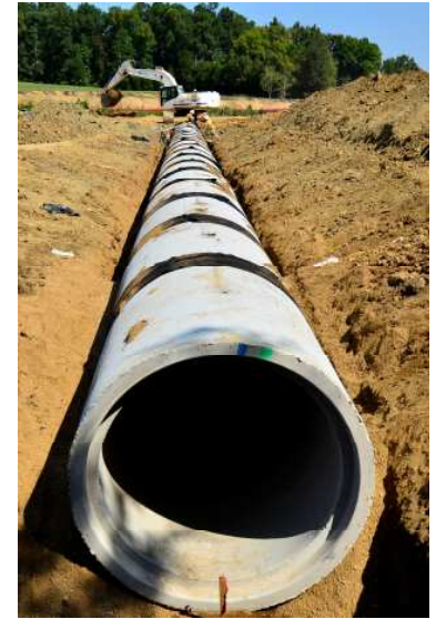
Pipe Installation: I-485 Charlotte Outer Loop
