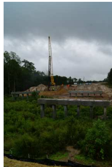
Linear Construction: Wilmington Bypass
