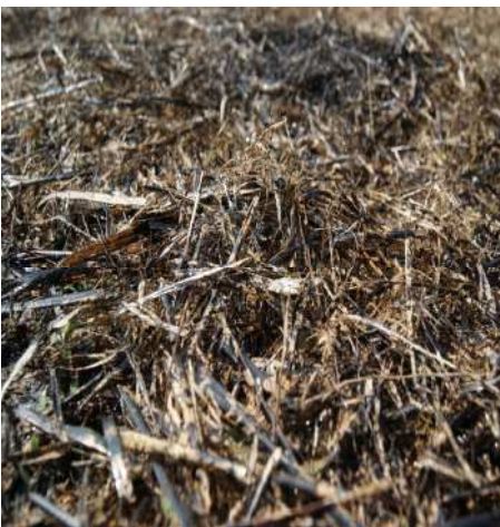
Straw: The Department is evaluating how well straw mulch works with turbidity reduction.
