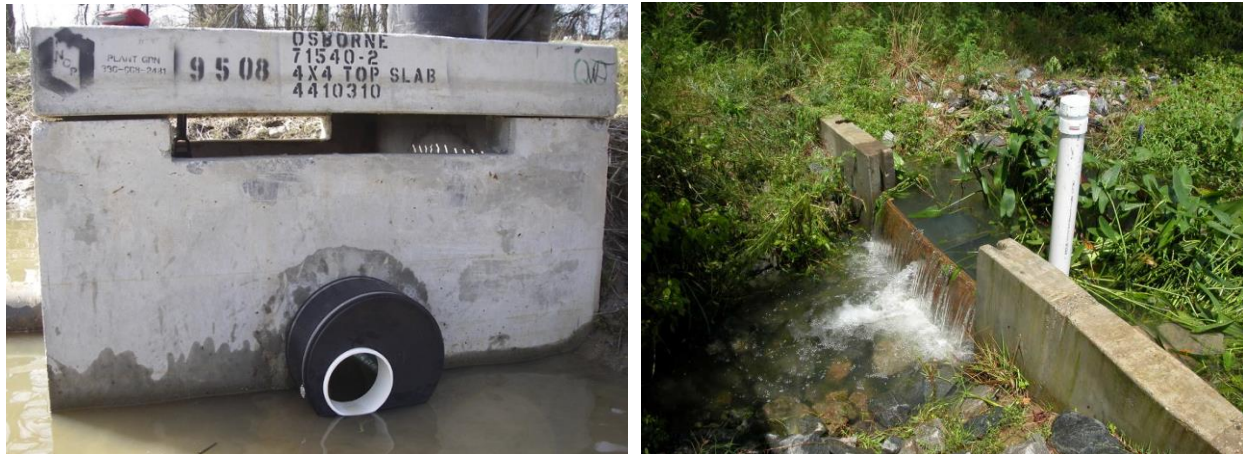
Figure 4: Two Examples of Adjustable Outlets
