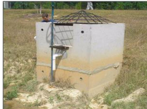
Figure 7: Outlet Structure
