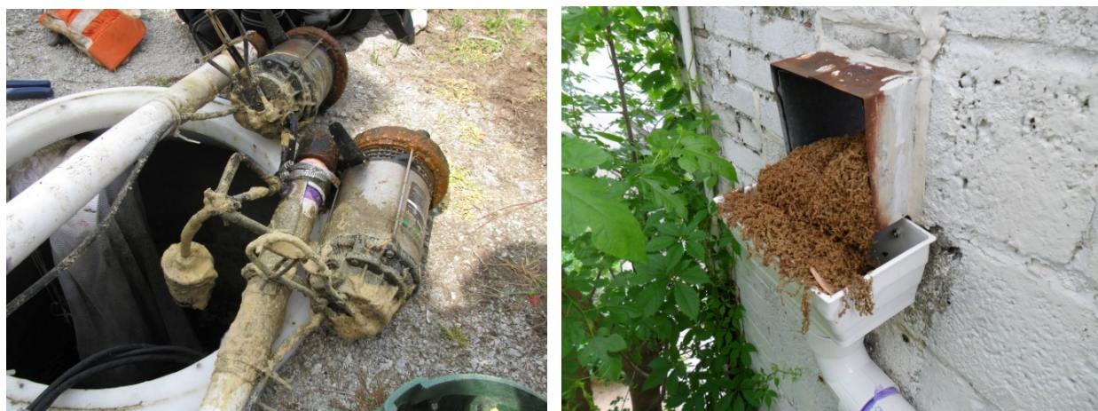
Figure 15. Pumps need to be pulled periodically for cleaning and preventive maintenance (left). Overhanging vegetation increases the needed frequency of maintenance (right) (NCSU BAE)
