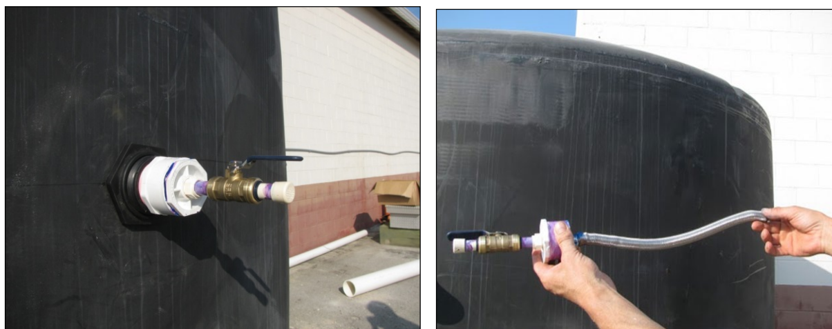
Figure 5. Anti-Clogging Passive Drawdown Mechanism (NCSU BAE)
