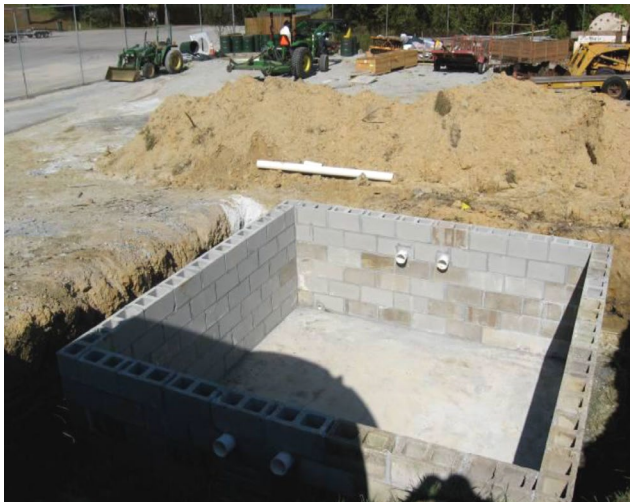
Figure 10. Preparing a cistern footing of aggregate (left) and a concrete footing for a cistern exceeding 1,500 gallons (right) (NCSU BAE)
