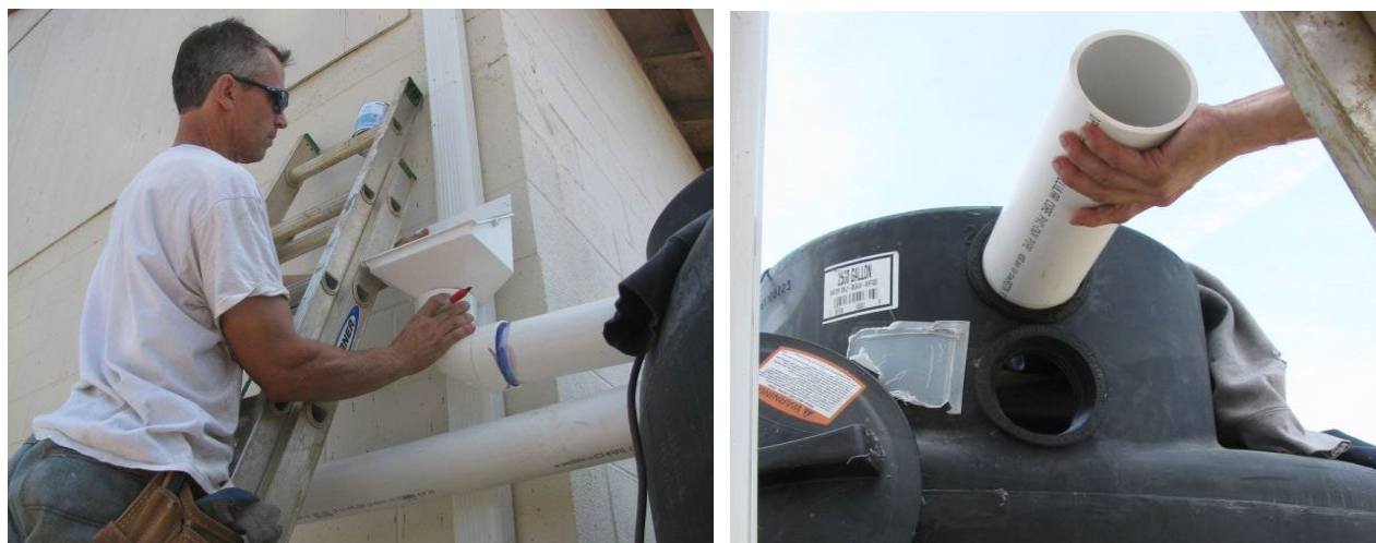
Figure 14. (a) Pipe leading from debris filter to the tank; (b) Rubber gasket used to create leak-free seal when pipe enters the tank. (NCSU-BAE)
