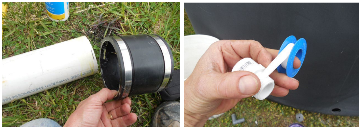
Figure 13. Ensure the connections are water-tight. (NCSU BAE)
