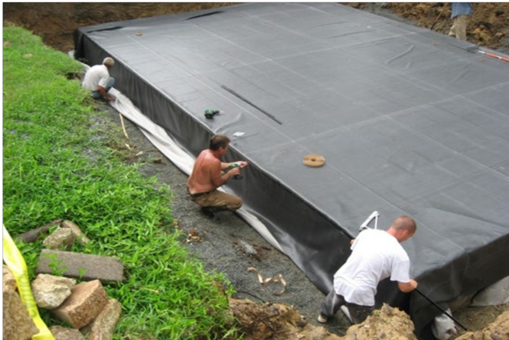
Figure 12. Installation of a membrane on a 15,000 gallon underground cistern at the Fayetteville Technical Community College NCSU BAE)
