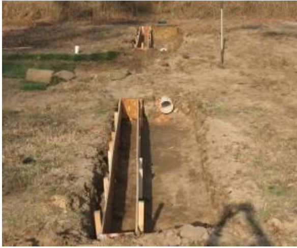
Figure 10: Forming the Level Lip (NCSU-BAE)
