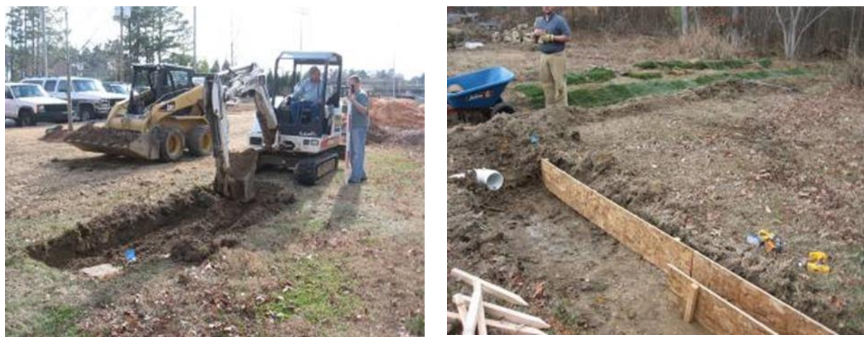
Figure 9: Excavating the Blind Swale (NCSU-BAE)
