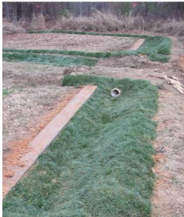
Figure 11: LS and Blind Swale Post-Construction
