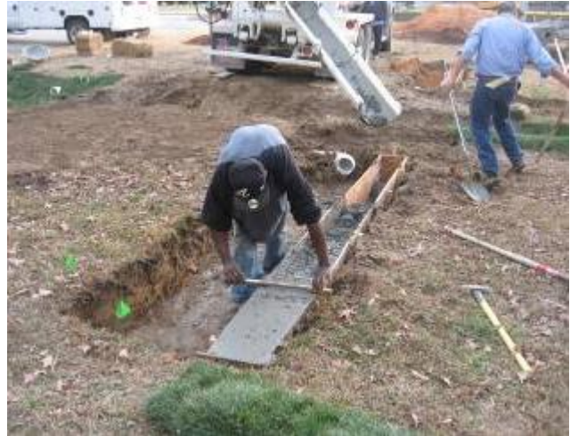
Figure 10: Forming the Level Lip (NCSU-BAE)
