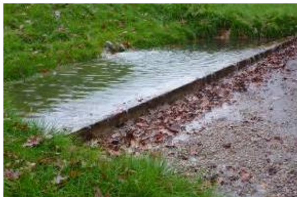
Figure 3: Level Spreader Lip (NCSU)
