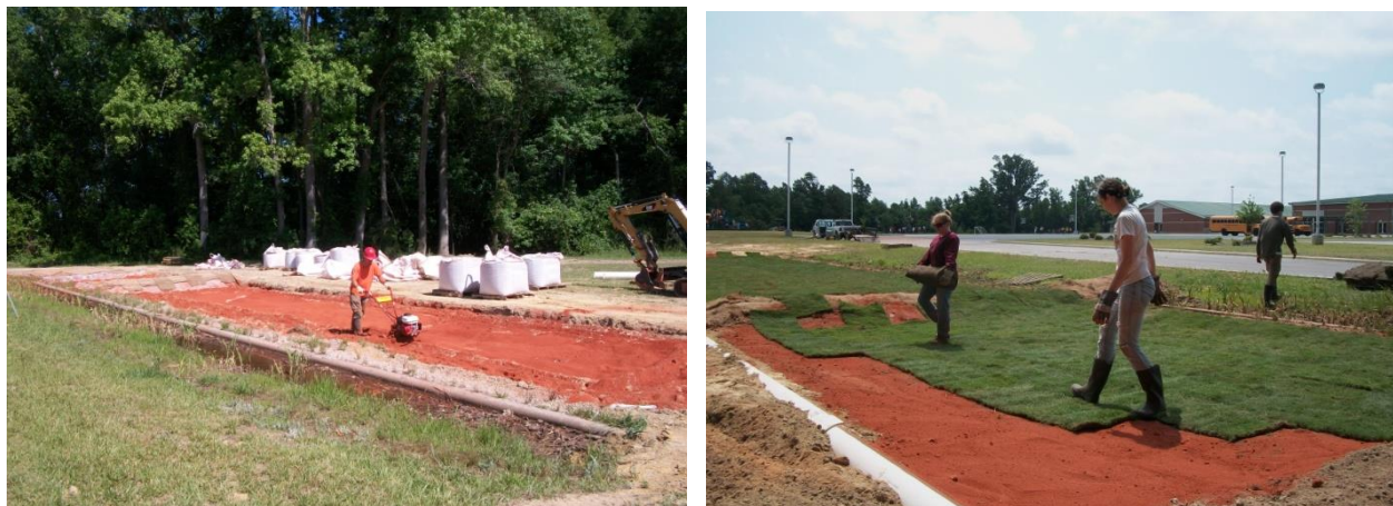
Figure 7: Installation of Soil Amendments
