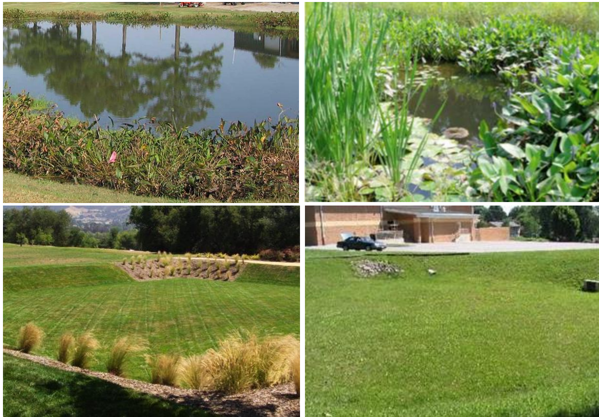
Figure 5: SCMs that Pond Water: Wet Pond (upper left), Stormwater Wetland (upper right), Infiltration Basin (lower left), and Dry Pond (lower right)
