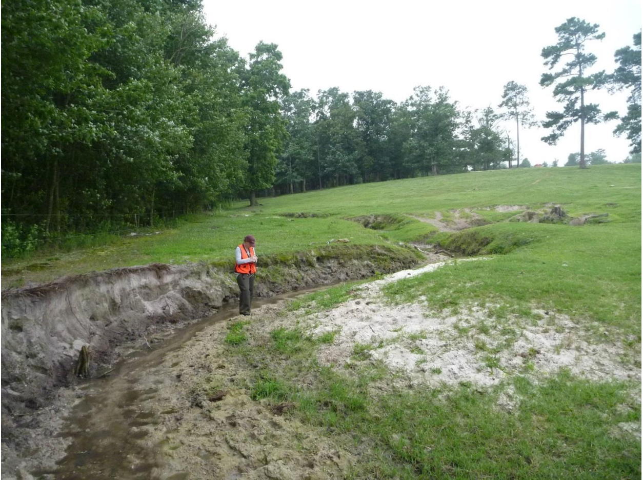
Figure 6. Bank erosion at potential stream restoration site WRO-051.
