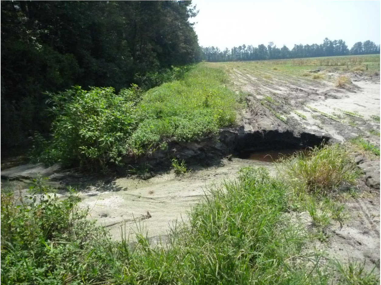
Figure 8. Headcut and erosion from an agricultural field in the LWP study area.
