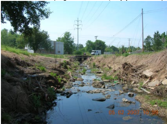
Figure 1: Stream Restoration Site in the Little Alamance Watershed
