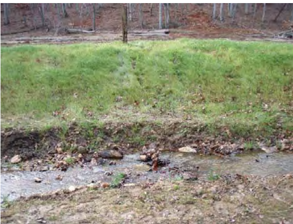
5.5d. Post-restoration riffle area.
