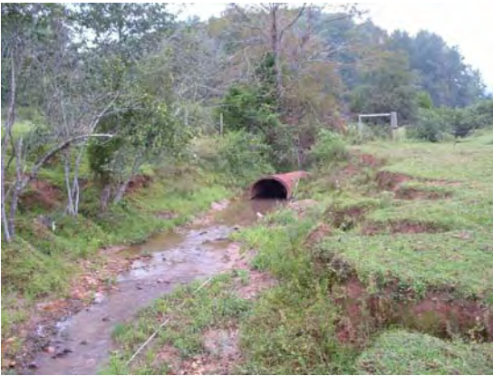
5.5b. Pre-restoration condition in straight section.
