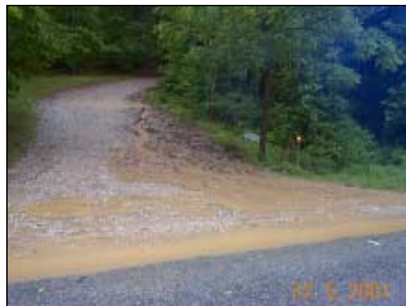
Figure 2.12 Runoff from gravel driveway in the upper Mud Creek watershed.
