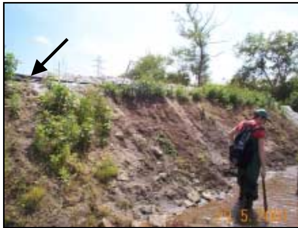
Figure 2.13 Scraped bank along Bat Fork. Note collapsed sediment fence.
