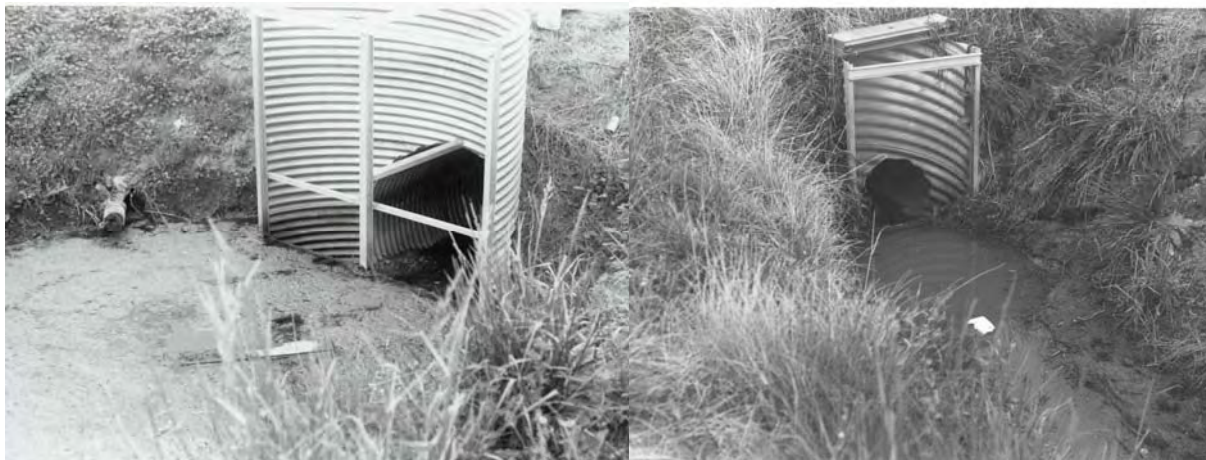
Exhibit 12. Flashboard risers with raised water level (left) and free drainage (right).
