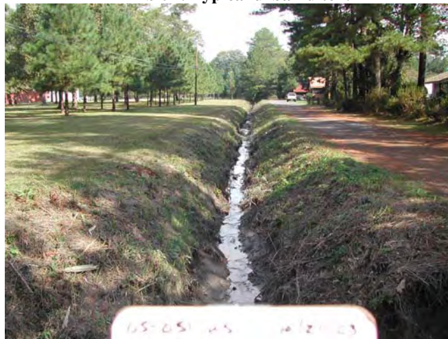
Exhibit 4. Typical urban ditch.
