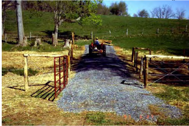
Exhibit 13. Cattle exclusion and stream crossing.
