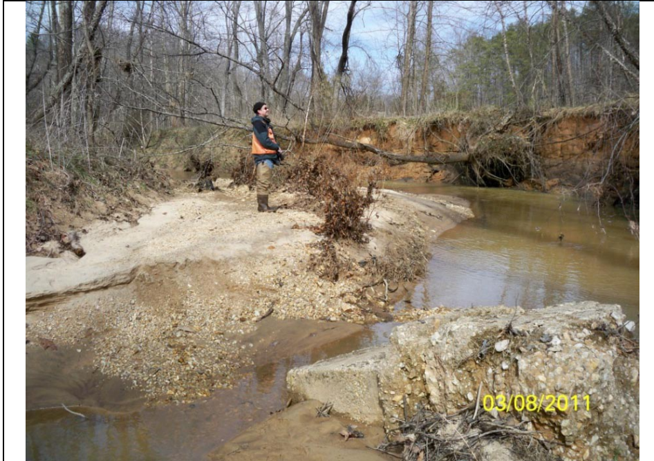
Photo 7. Chinquapin Creek at SR1830 (CH-1). Note the turbid conditions 40 hours following a storm event of approximately two inches over a less than 24-hour period. Also note the stream bank erosion and coarse material located along the inside bend of the meander. Drainage area at this point is 9.4 square miles.
