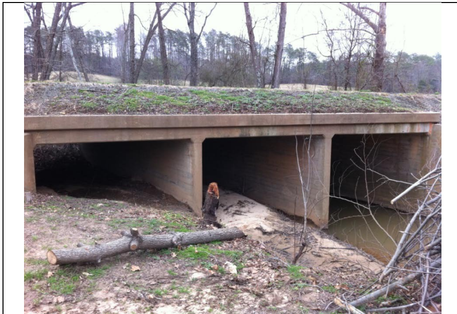
Photo 8. Chinquapin Creek at SR1809 (CH-2). Note the excessive sediment accumulation in the box culvert. The sediment is a likely stressor to habitat functions in Chinquapin Creek and other streams in the planning area.
