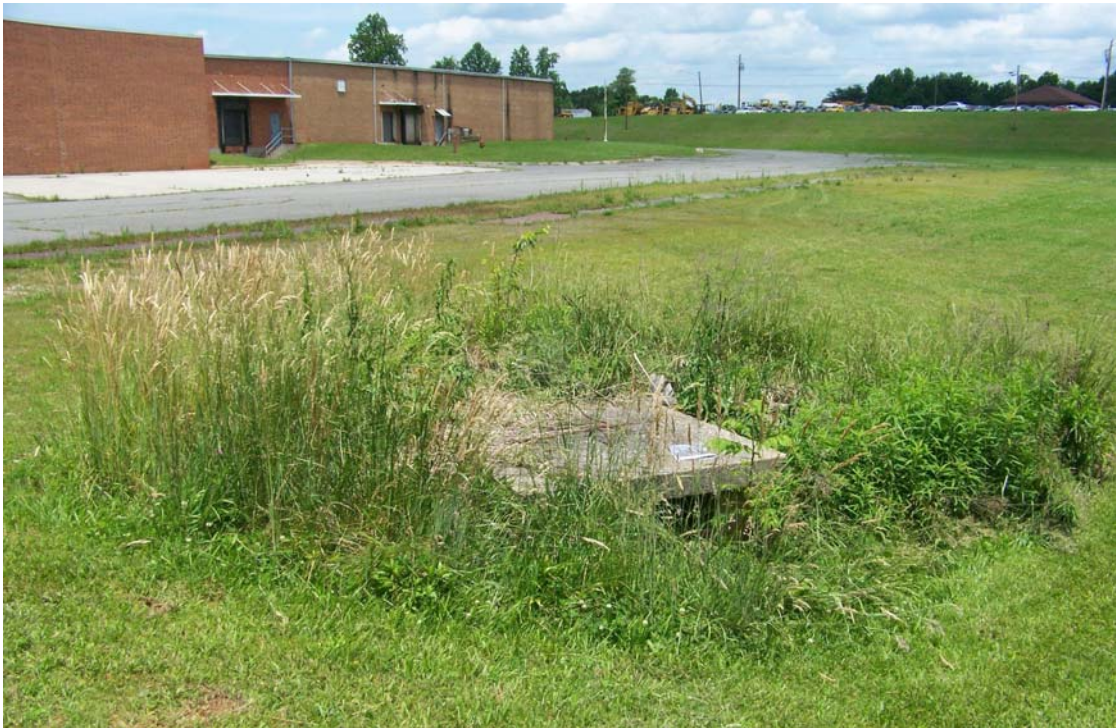
BMP Site 2. Existing site and outlet structure.
