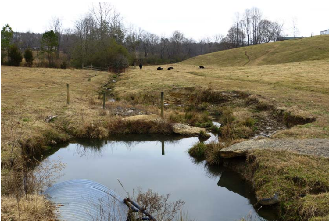
Wetland Site W9. Bank erosion related to livestock access along UT to Toms Creek.
