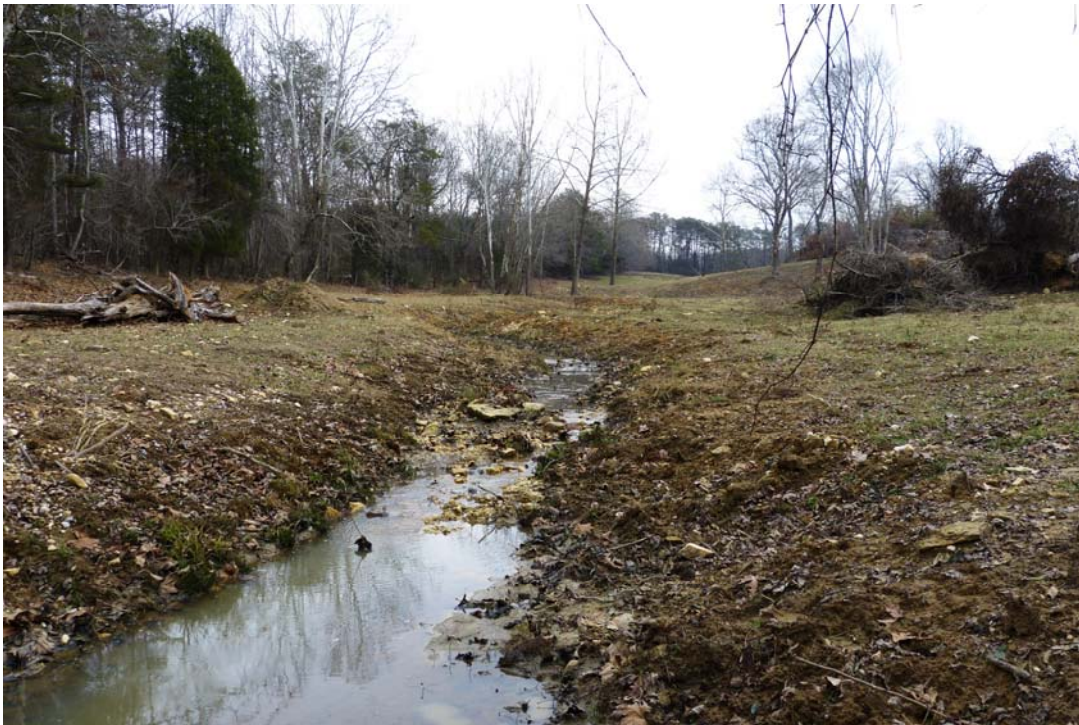
Stream Site P32. Stream banks in poor condition along UT to Chinquapin Creek due to livestock access.
