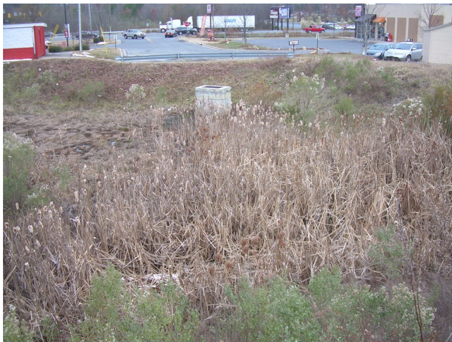
Site 5, looking across toward outlet
