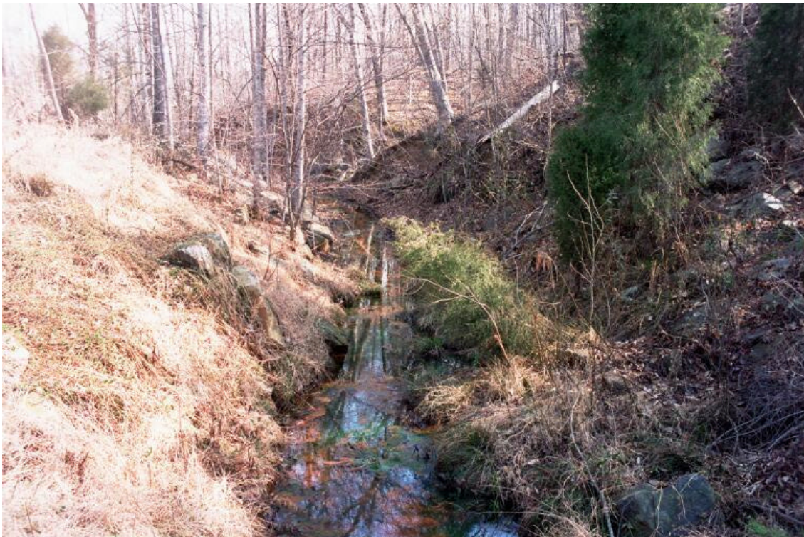
32. Ash Pond Dam. Outlet channel from east weir. Minor obstruction, not significant.
