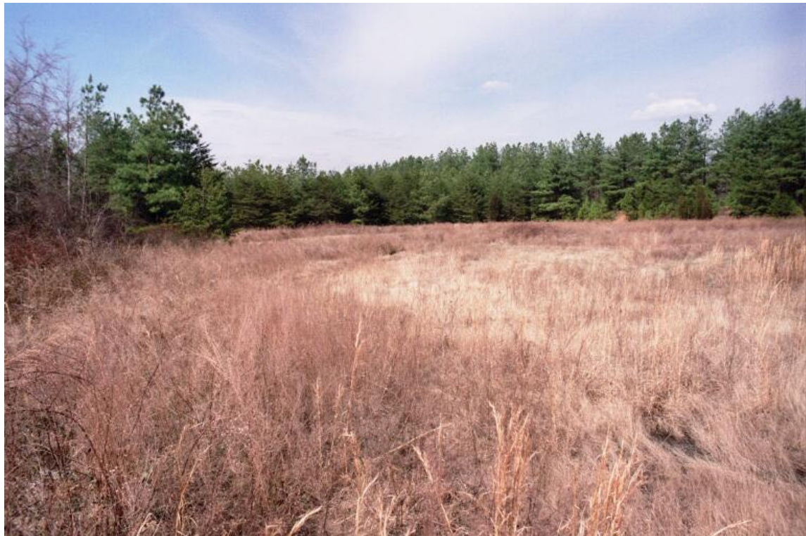
20. Mayo Creek Dam. East side of emergency spillway. Trees in spillway cut after field visit.
