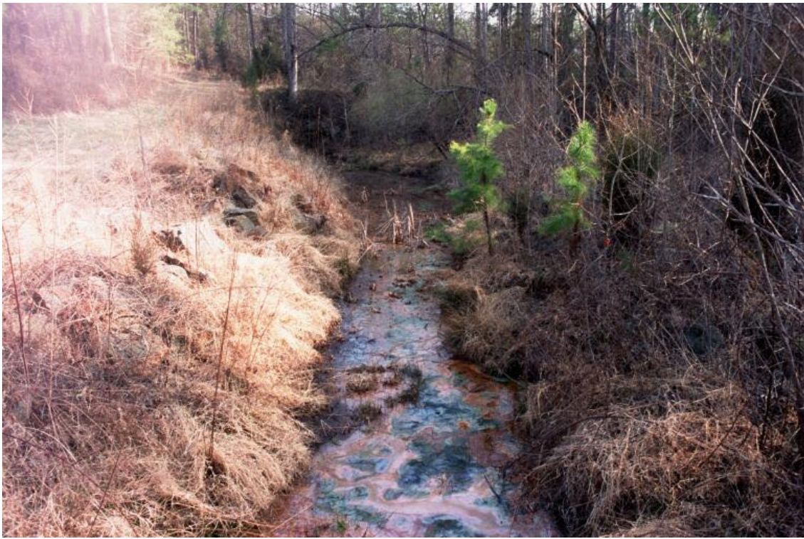
31. Ash Pond Dam. Outlet channel from west weir. No obstructions.
