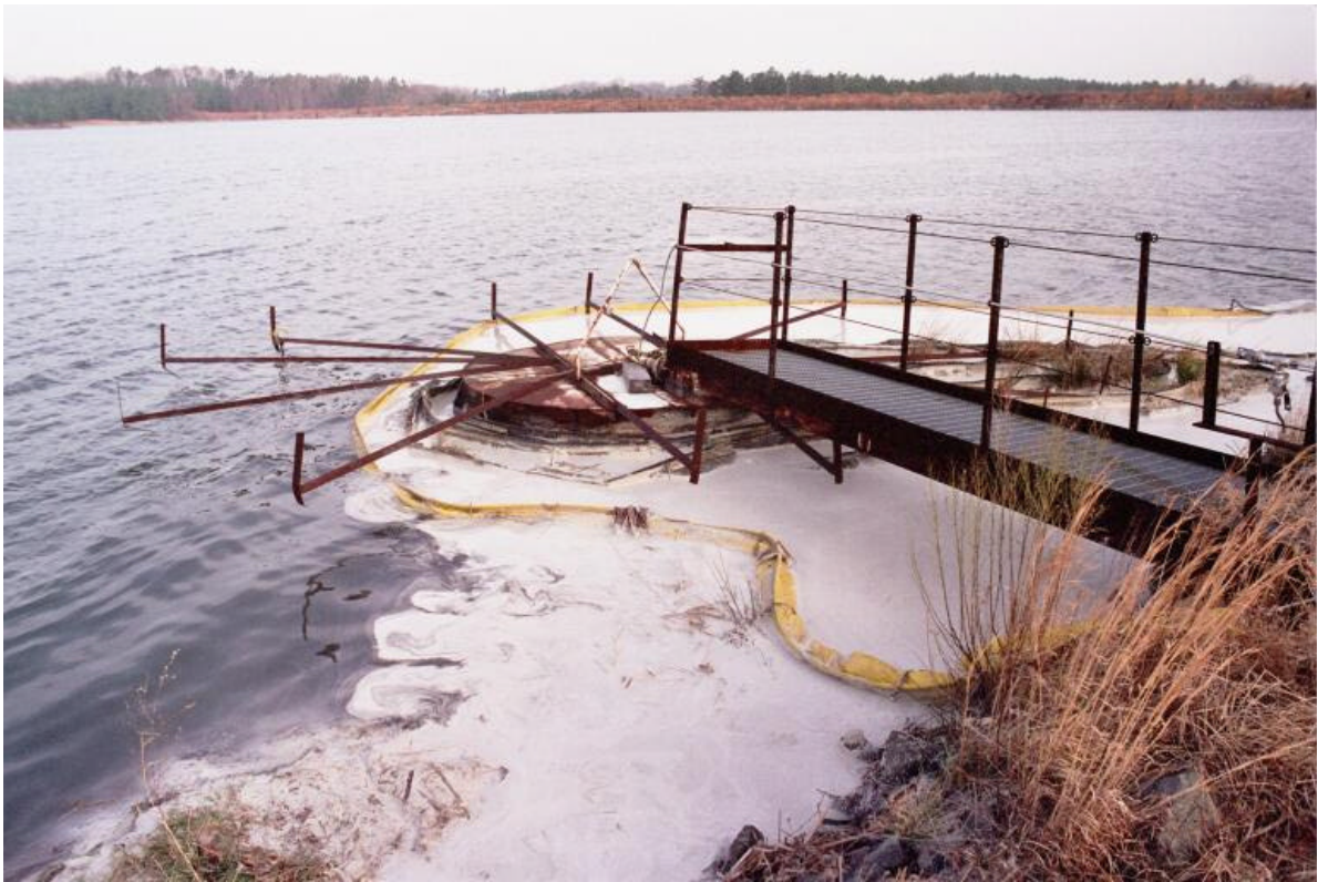
33. Ash Pond Dam. Skimmer at pond outlet structure.
