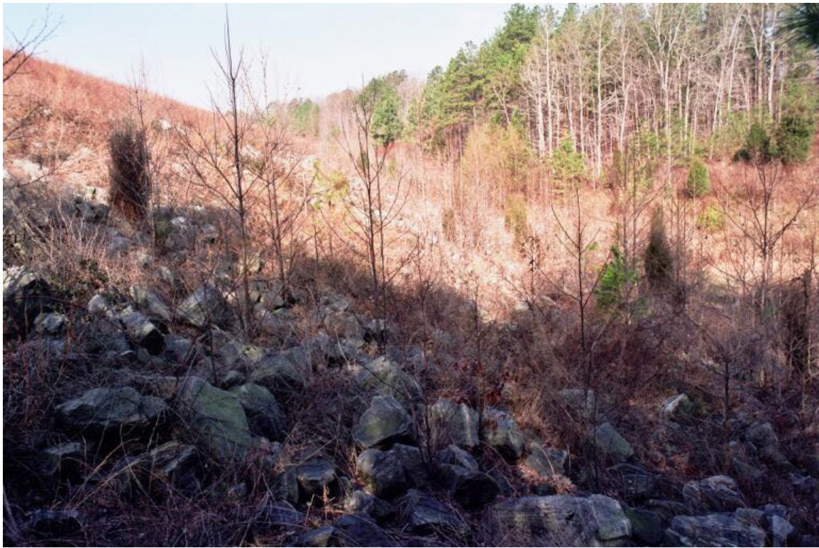
25. Ash Pond Dam. Downstream slope of west section. Note some trees still alive.
