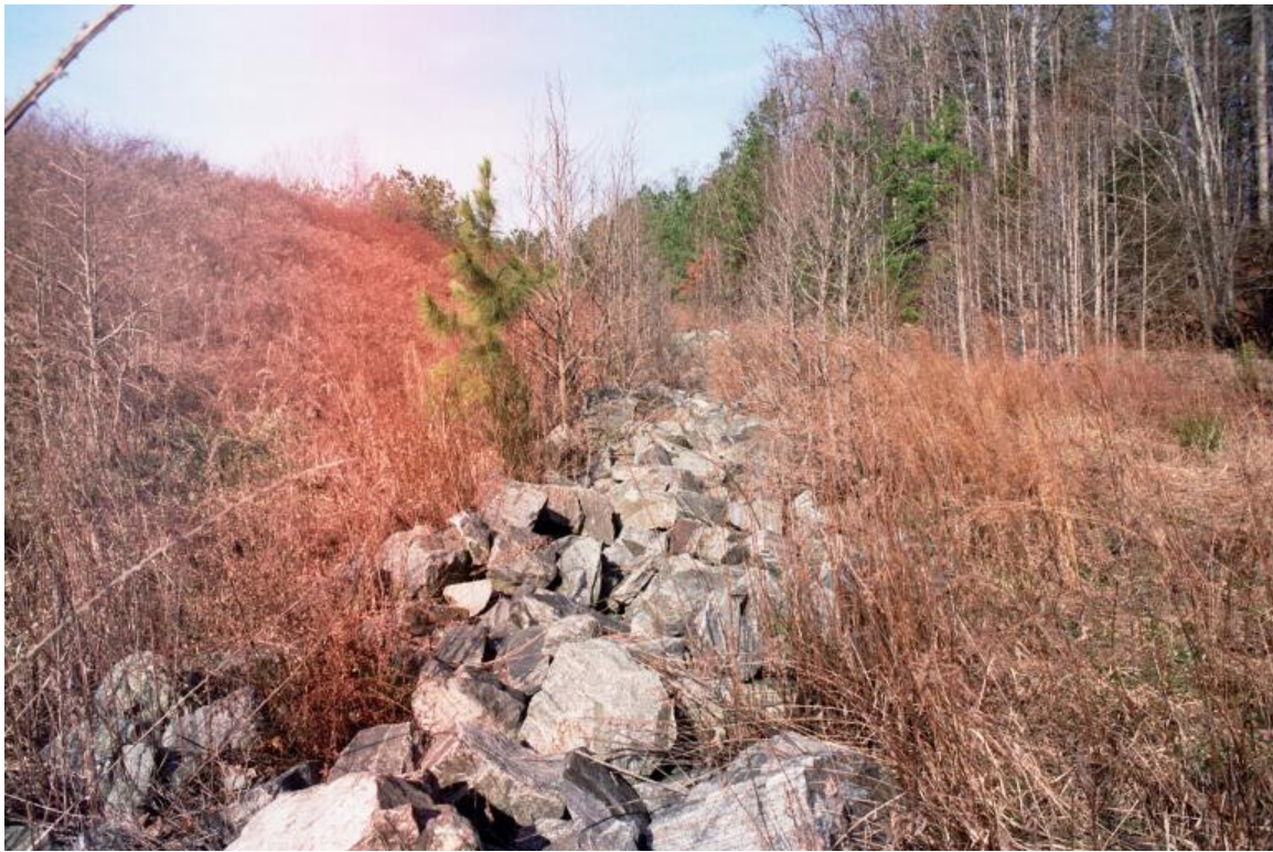
26. Ash Pond Dam. Rock toe along west section. Note some trees need cutting or spraying.
