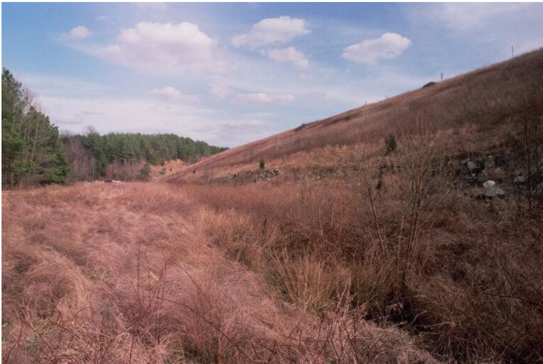
5. Mayo Creek Dam. Downstream slope looking east from west end.
