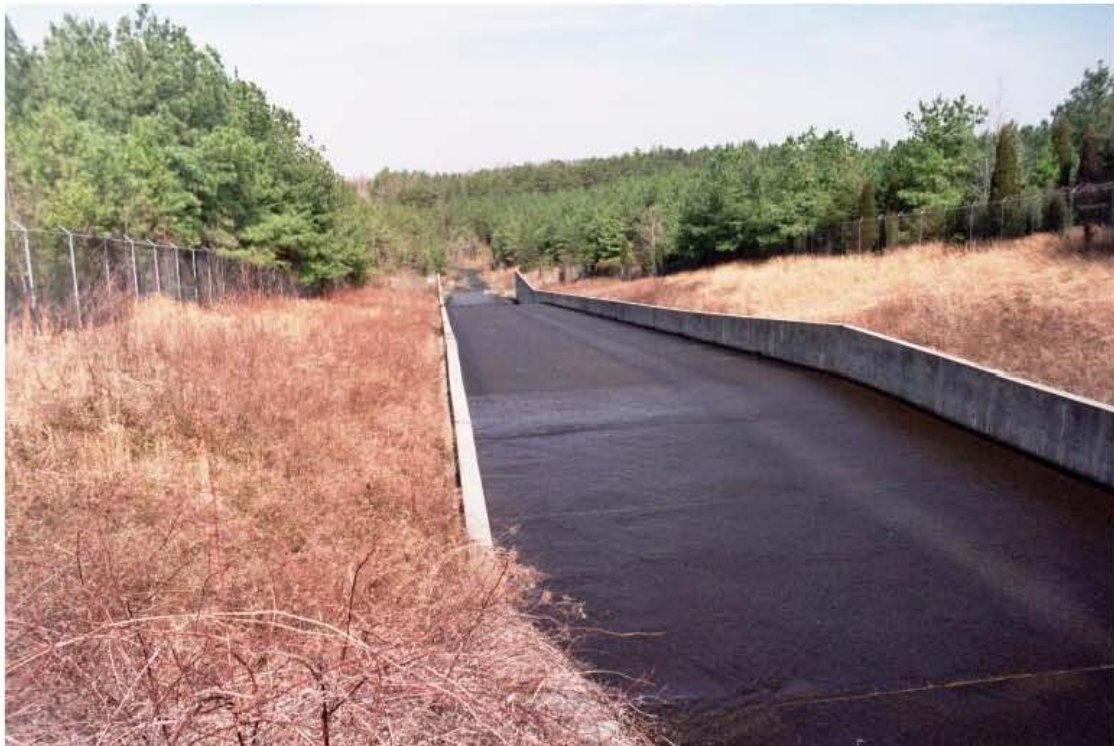
14. Mayo Creek Dam. Primary spillway looking downstream from near ogee section. Note smooth flow of water.
