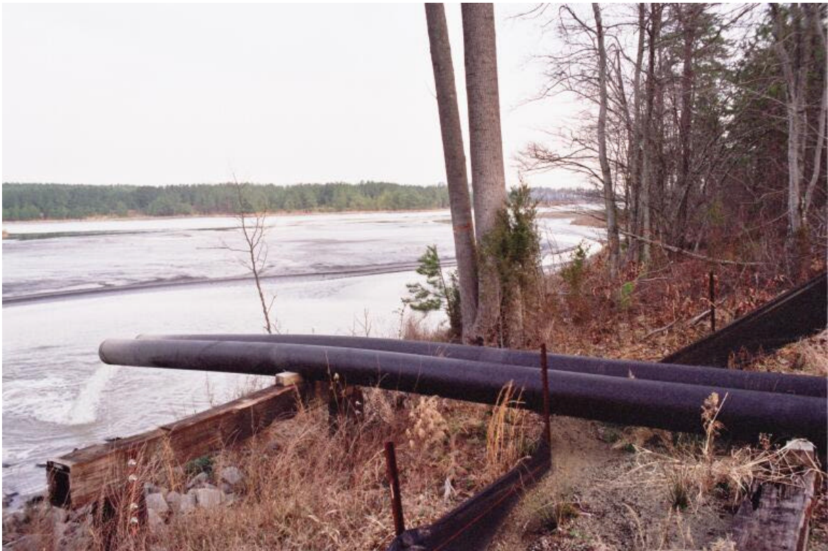
36. Ash Pond Dam. Discharge of extended fly ash lines.
