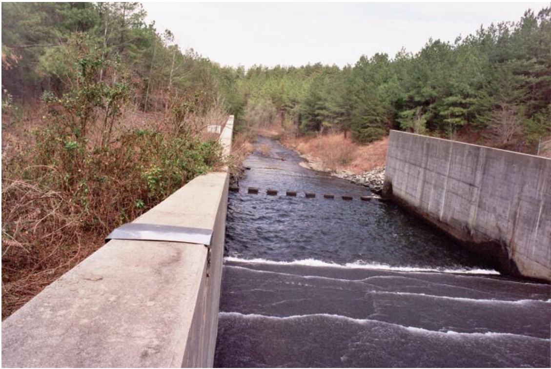
15. Mayo Creek Dam. Discharge end and outlet channel of Primary spillway. Note no flow obstructions.
