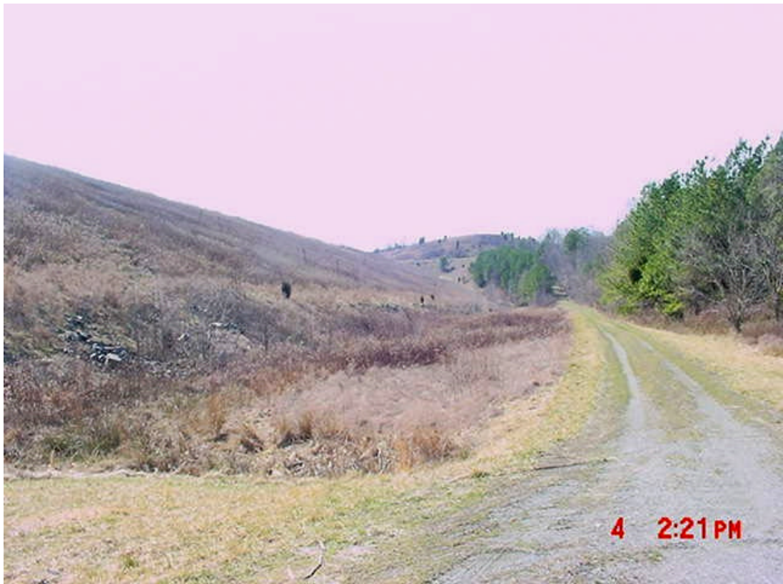
6. Mayo Creek Dam. Downstream slope looking west from discharge stilling basin.
