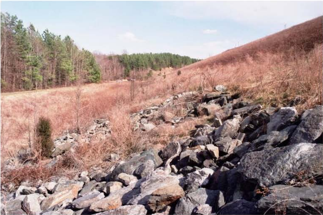
8. Mayo Creek Dam. General view of rock toe.
