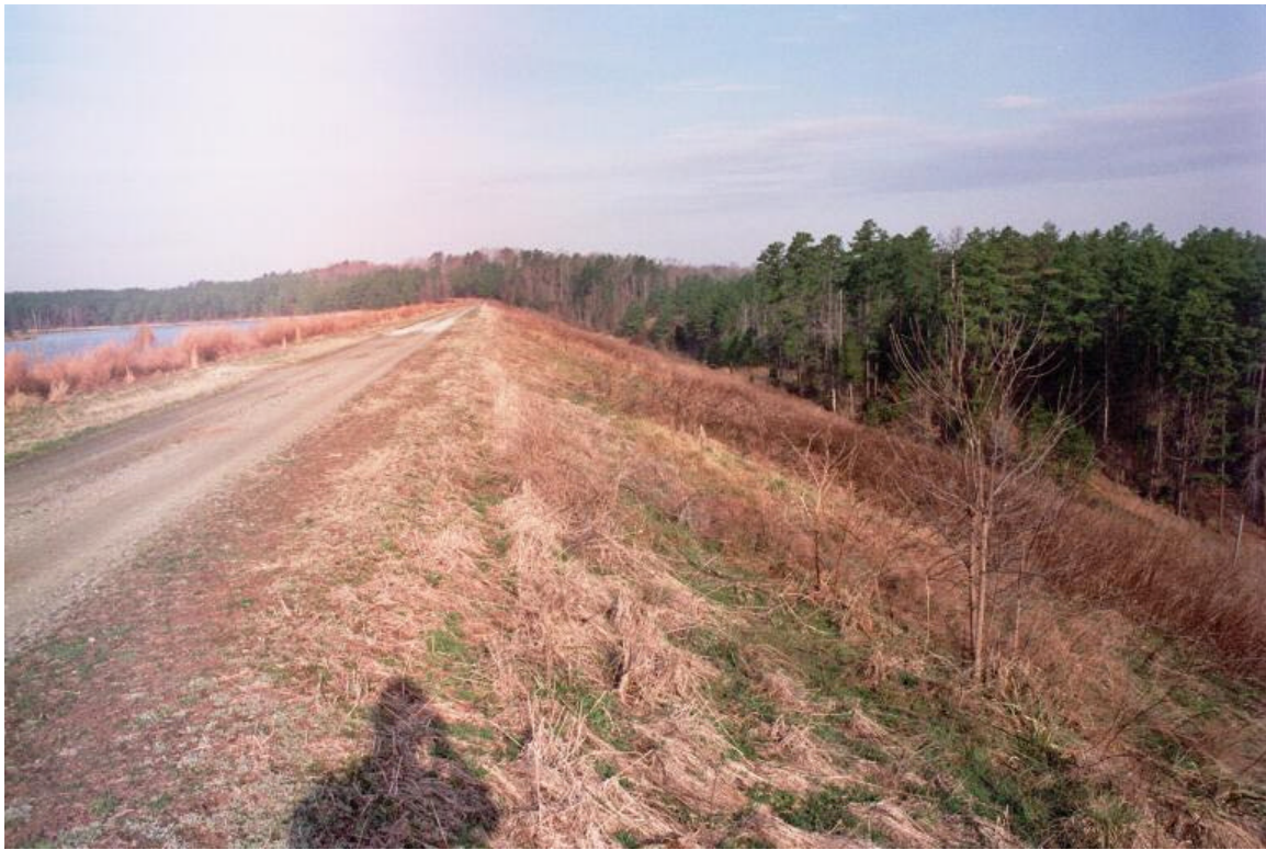
21. Ash Pond Dam. Crest and downstream slope. Note scattered small trees.
