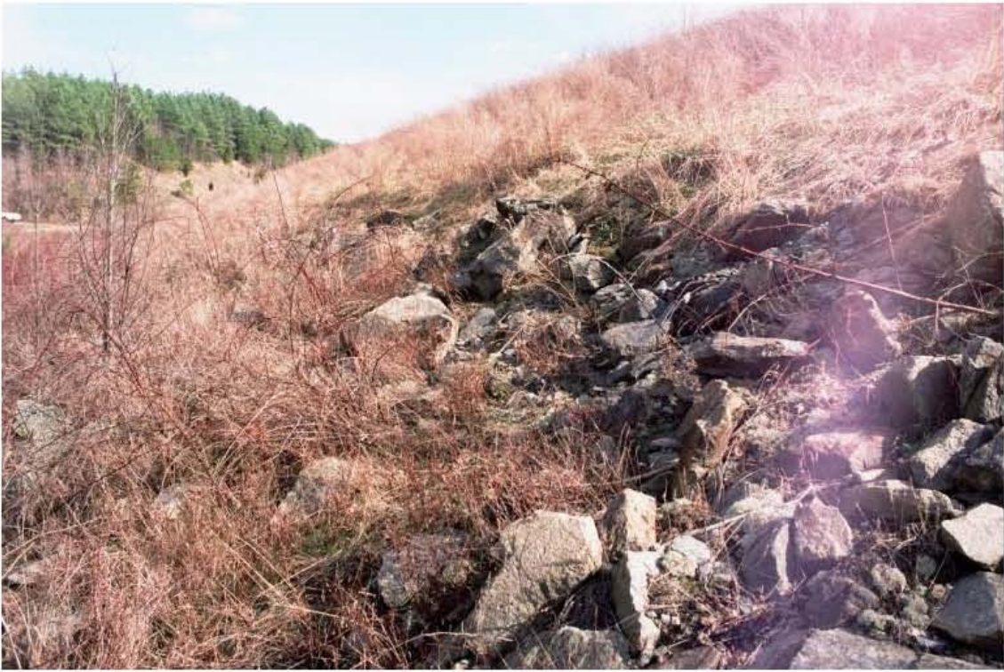
7. Mayo Creek Dam. Rock toe in area noted as disturbed in 1994. No apparent change.
