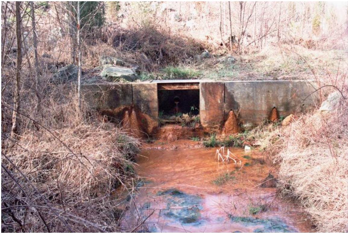
29. Ash Pond Dam. West weir. Note sediment accumulation at weep holes. No impact on dam.
