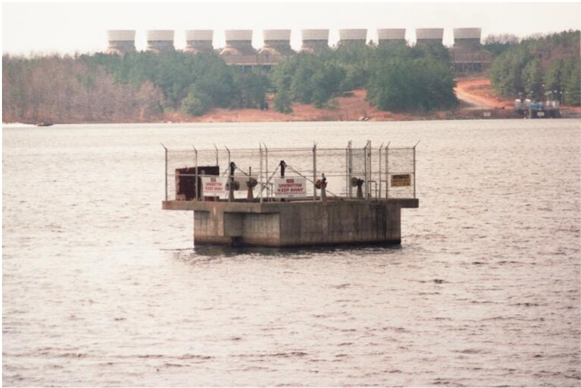
11. Mayo Creek Dam. Outlet structure in lake.
