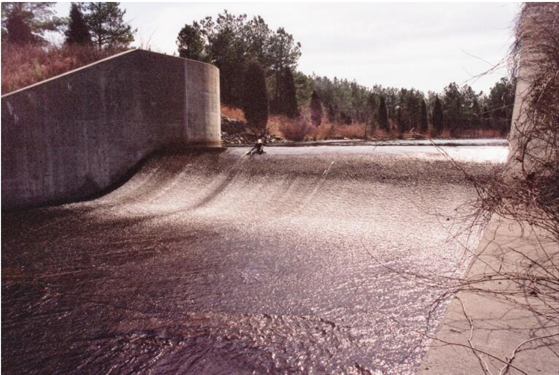
17. Mayo Creek Dam. Ogee section of primary spillway. Note smooth flow pattern.
