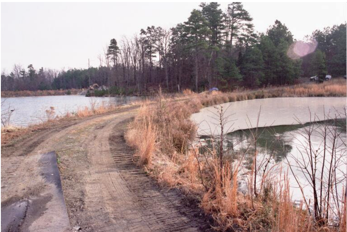
34. Ash Pond Dam. Crest and downstream slope of secondary pond. Small trees need controlling.
