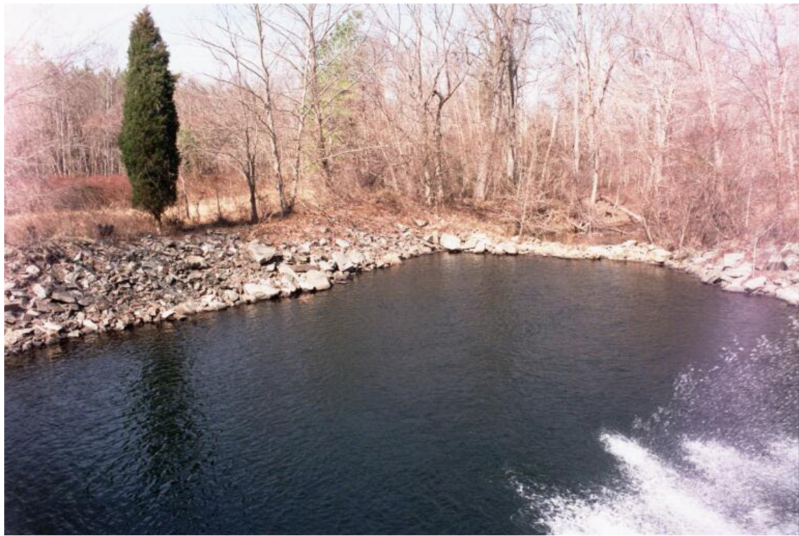
12. Mayo Creek Dam. Stilling basin for outlet discharge.
