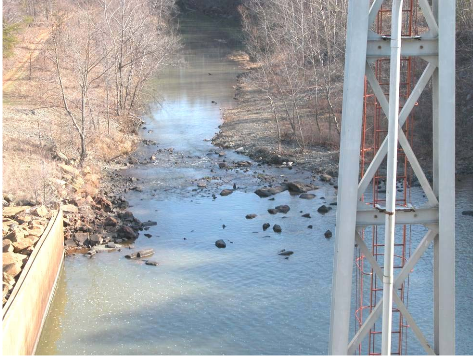
68. Afterbay Dam – View of downstream channel, no major obstructions.
