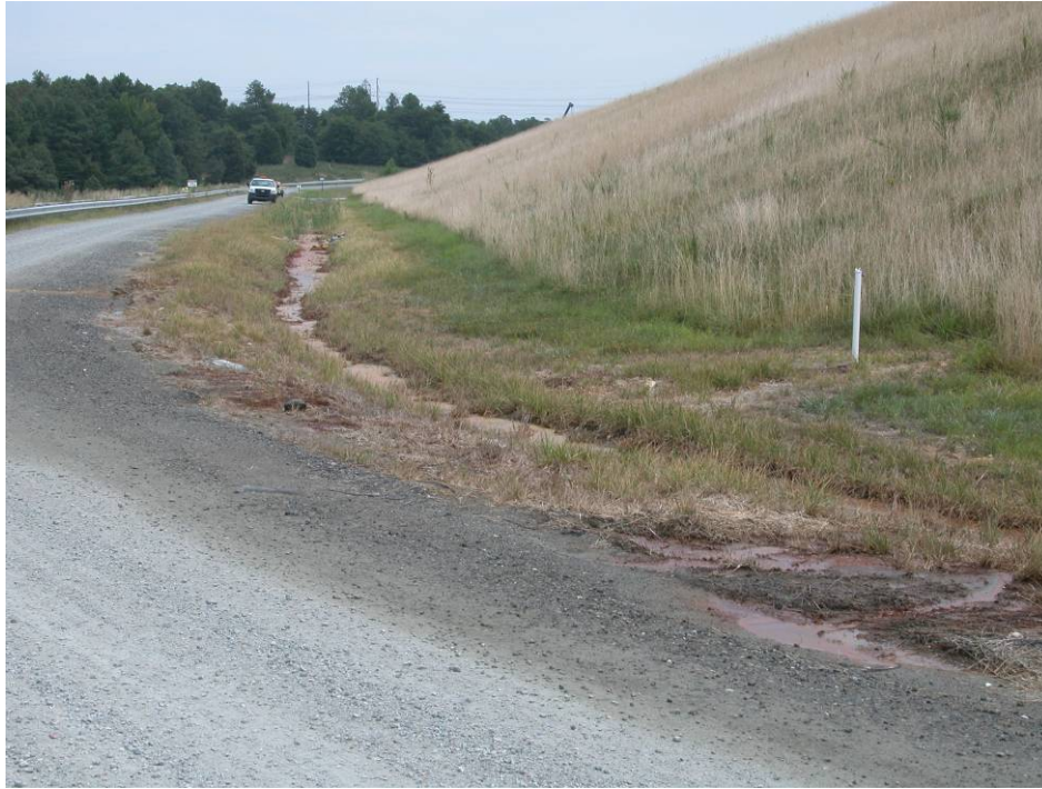
27. West Ash Pond Dam – View along crest of dam from west abutment. Toe of slope and drainage swale for new wastewater treatment pond is to the north (August 5, 2008)
