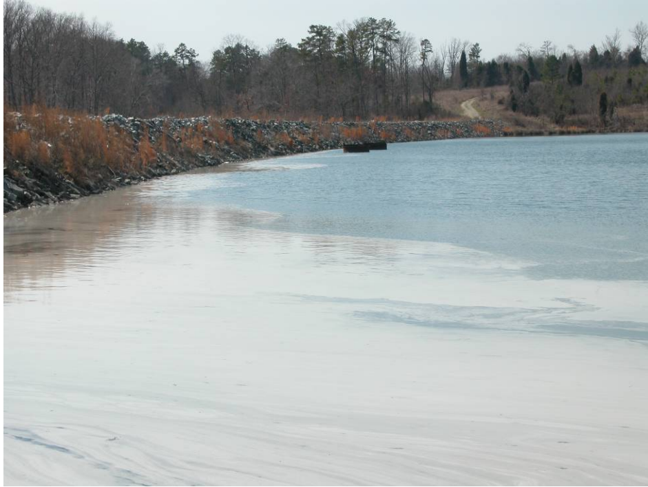
31. West Ash Pond Dike No. 1 – Interior slope looking toward west abutment.
