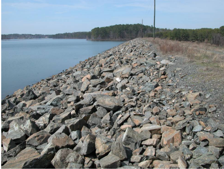
1. Main Dam – Crest and upstream slope looking west.
