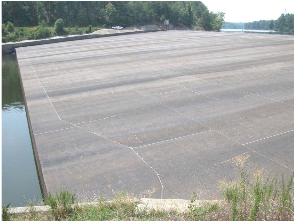
10. Main Dam – Lower spillway from left wall (August 5, 2008).
