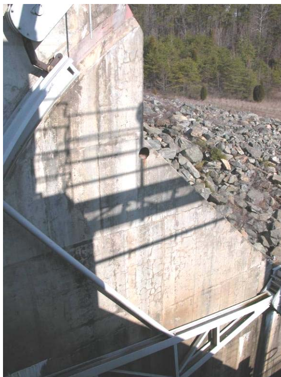
43. Afterbay Dam – West side Pier 1.
