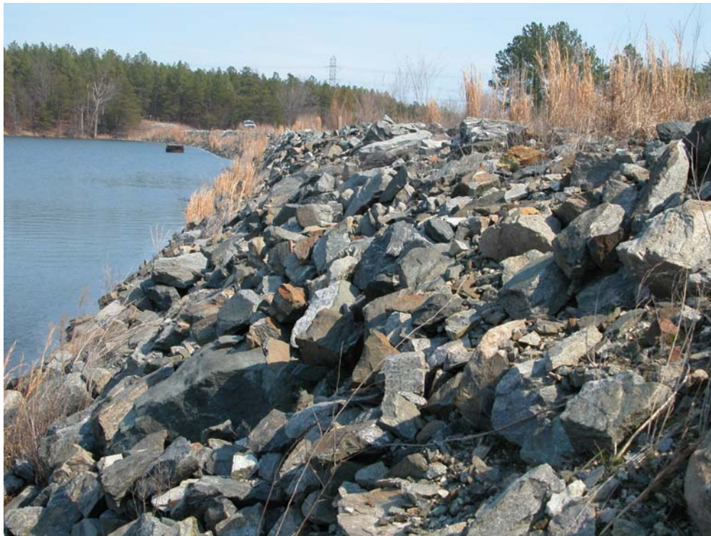
32. West Ash Pond Dike No. 1 – Rip rap on interior slope
