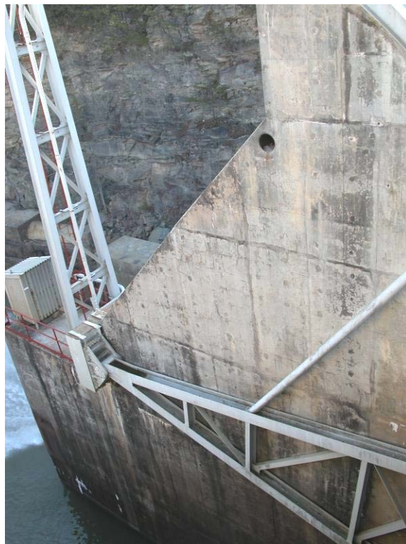
48. Afterbay Dam – East side Pier 4.
