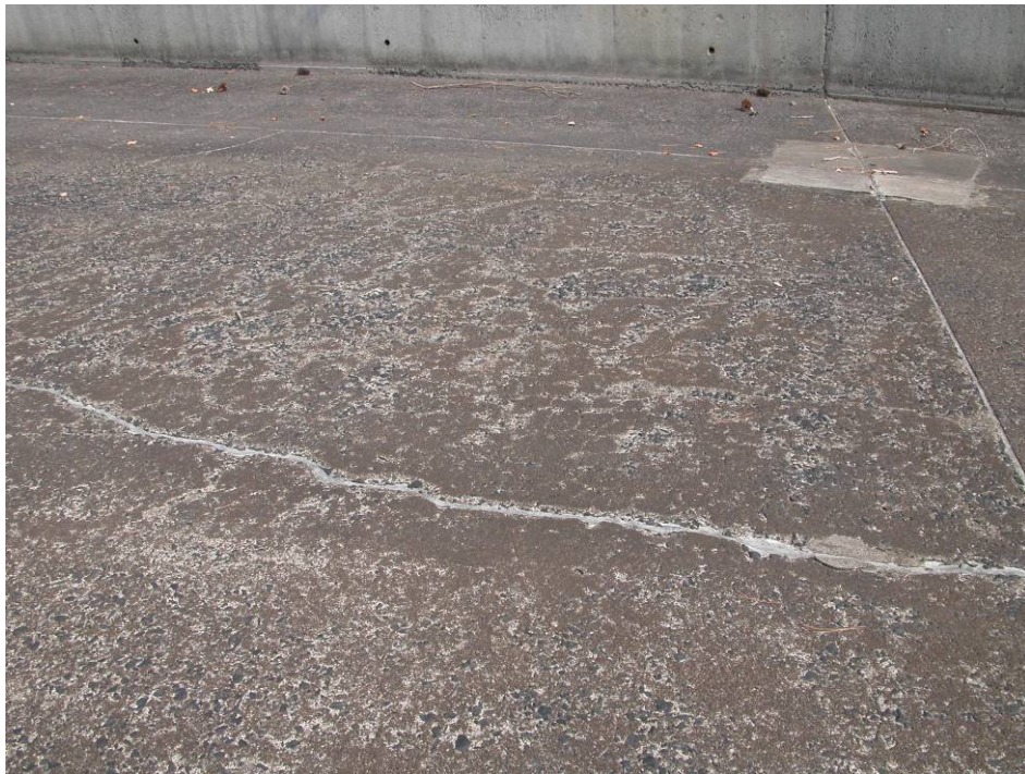
26. Exposed aggregate in section C12 (August 5, 2008).
