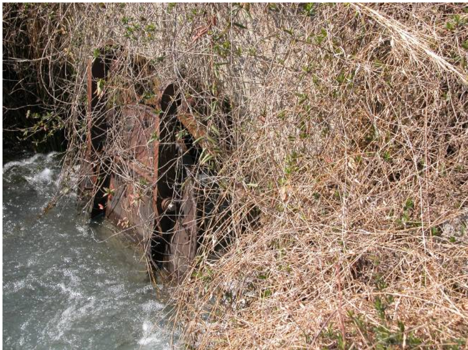
37. West Ash Pond Dike No. 1 – East flap gate.
