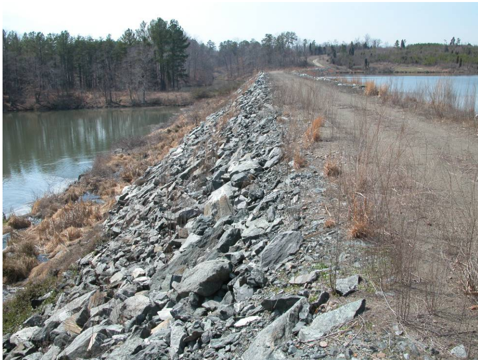
30. West Ash Pond Dike No. 1 – Crest and exterior slope looking toward west abutment.
