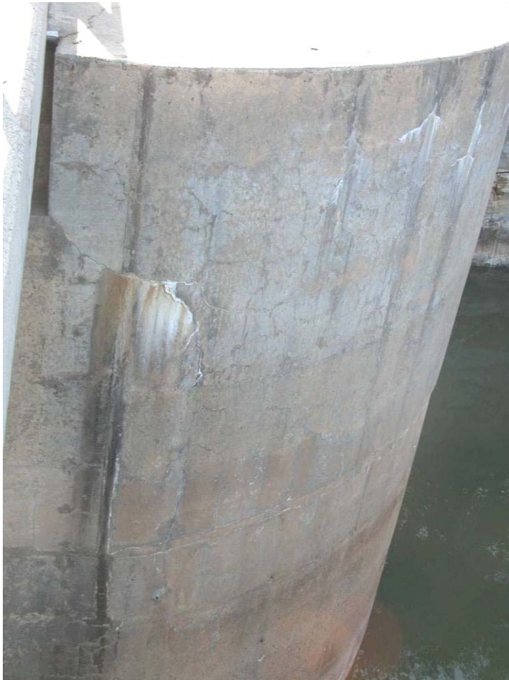
60. Afterbay Dam – East side Pier 5, upstream.
