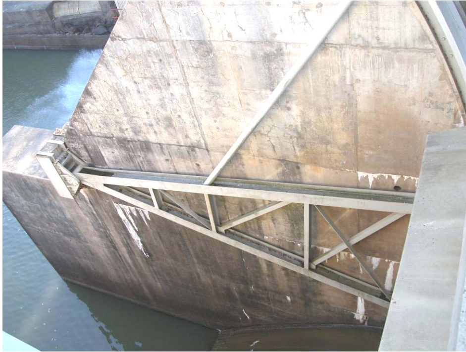
46. Afterbay Dam – East side Pier 3.
