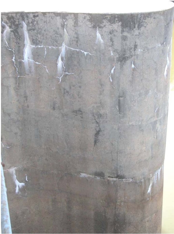
52. Afterbay Dam – East side Pier 1, upstream.
