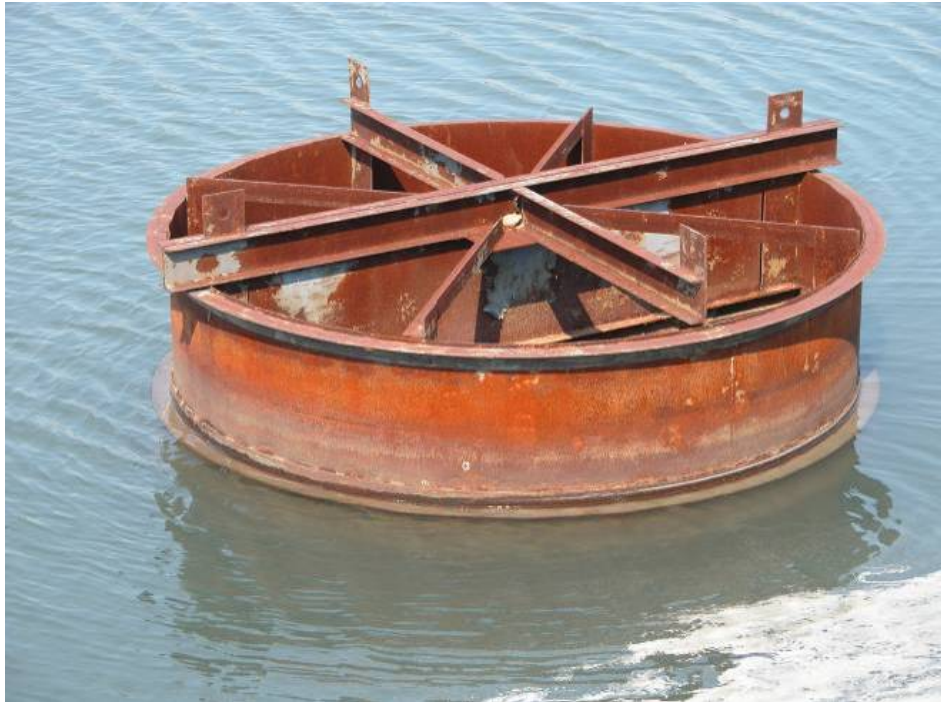
35. West Ash Pond Dike No. 1 – East skimmer.
