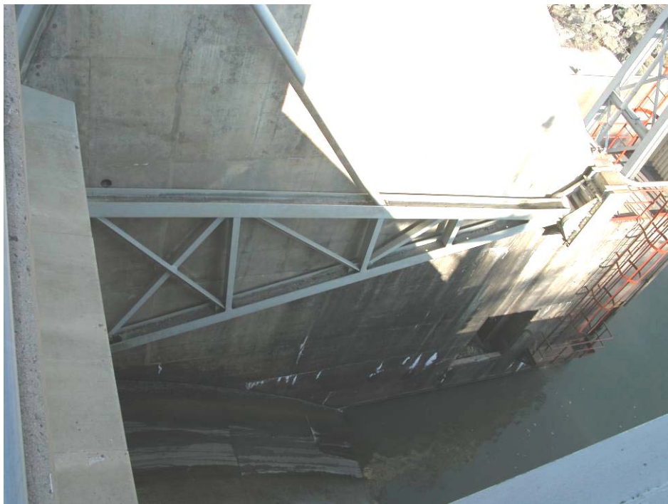
45. Afterbay Dam – West side Pier 2.
