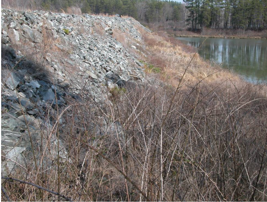
33. West Ash Pond Dike No. 1 – Riprap and toe of exterior slope looking toward east.
