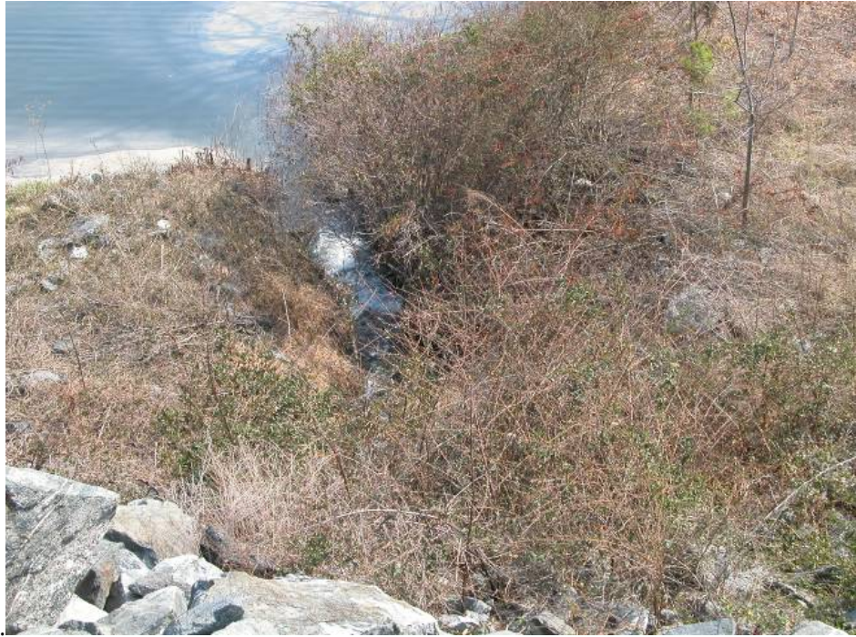
39. West Ash Pond Dike No. 1 – East outflow channel.
