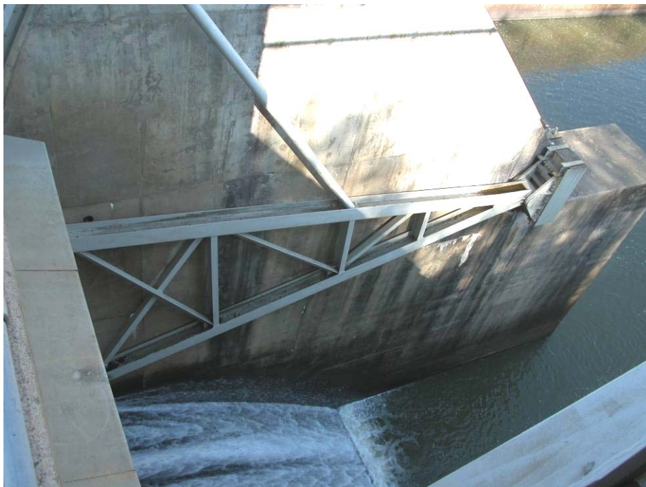
47. Afterbay Dam – West side Pier 3.
