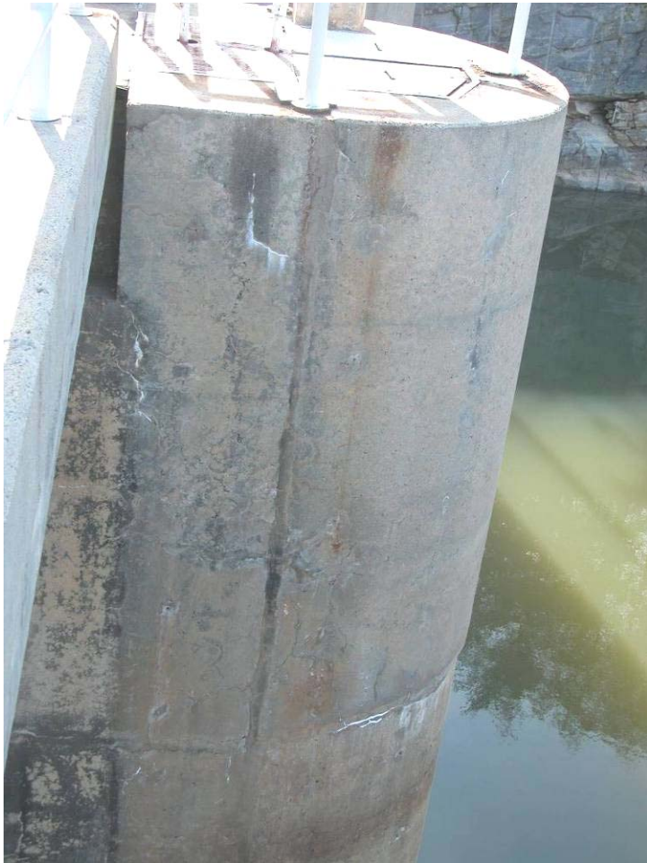
58. Afterbay Dam – East side Pier 4, upstream.
