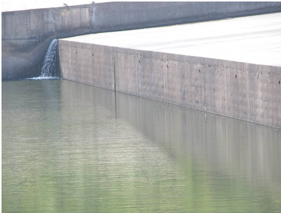
11. Main Dam – Drop wall (August 5, 2008).
