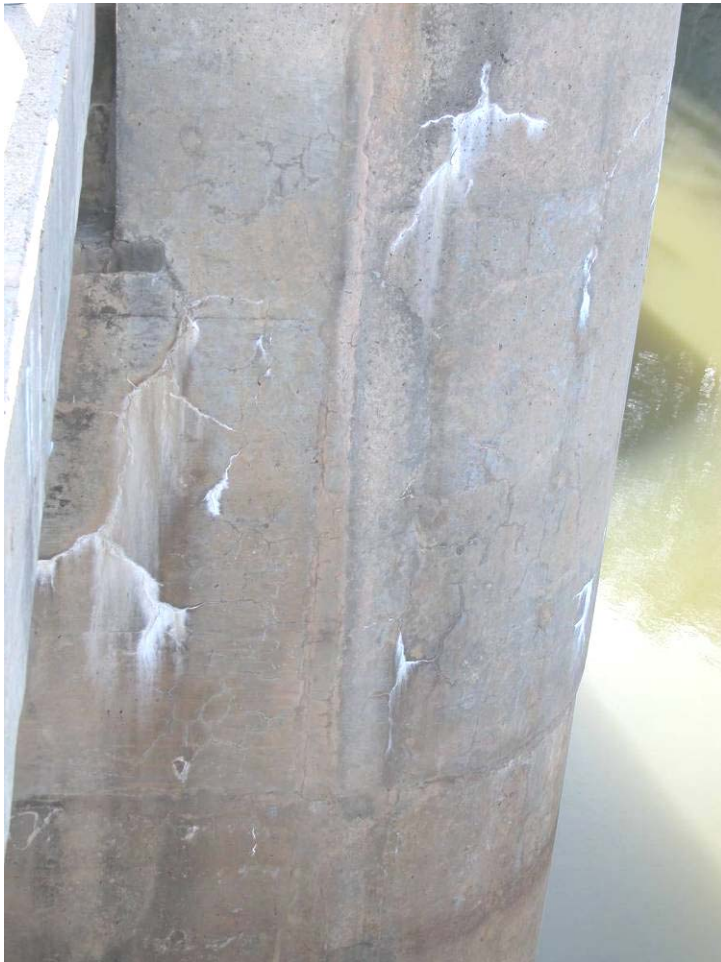
56. Afterbay Dam – East side Pier 3, upstream.
