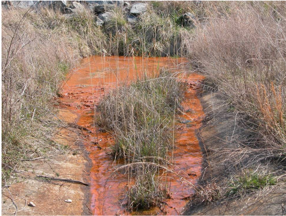
29. West Ash Pond Dam – Typical condition of toe drain outflow channels where flow is present.
