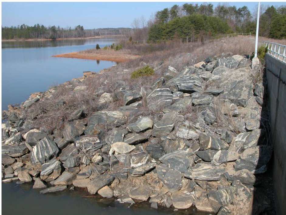
69. Afterbay Dam – View of upstream slope earth embankment section.
