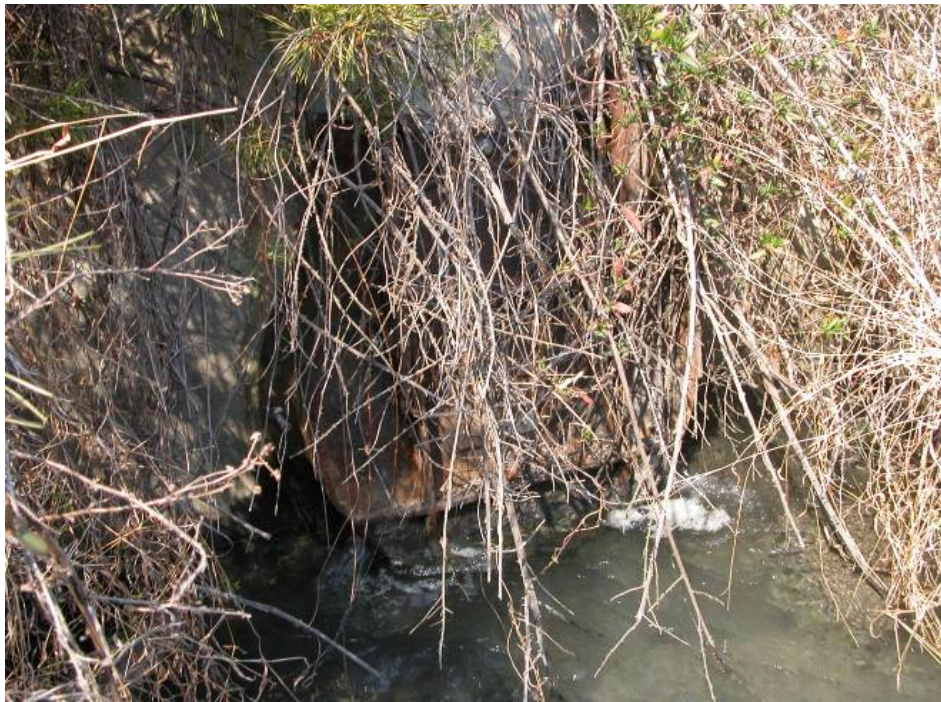
36. West Ash Pond Dike No. 1 – West flap gate.
