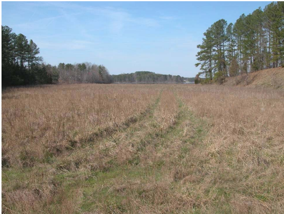
6. Main Dam – Emergency spillway looking toward lake.
