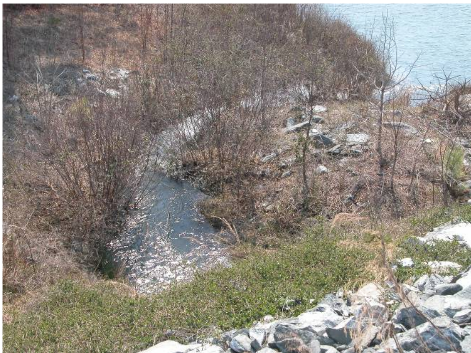
38. West Ash Pond Dike No. 1 – West outflow channel.
