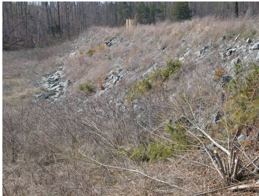
41. West Ash Pond Dike No. 4 – Exterior slope.
