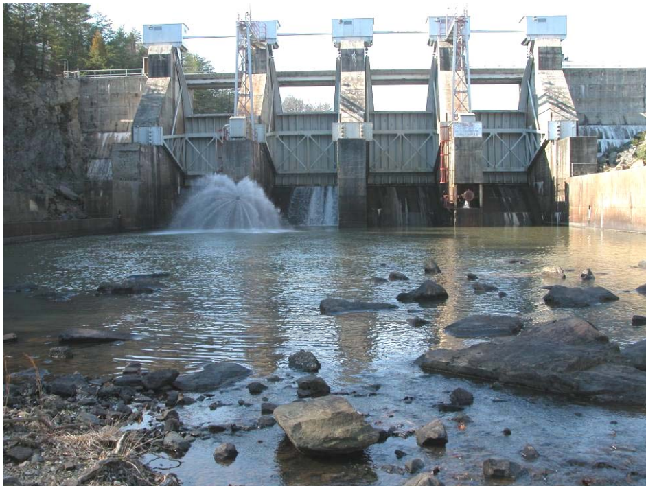
67. Afterbay Dam – General view of downstream concrete section.
