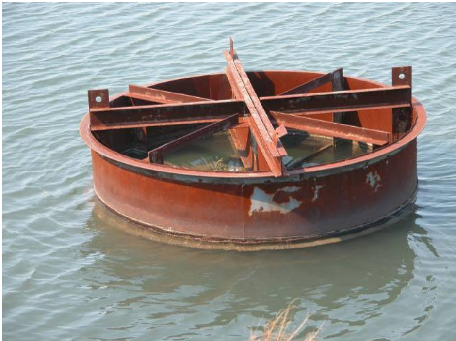
34. West Ash Pond Dike No. 1 – West skimmer.
