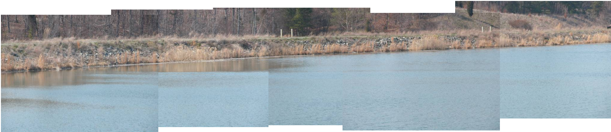
40. West Ash Pond Dike No. 4 –Interior slope.
