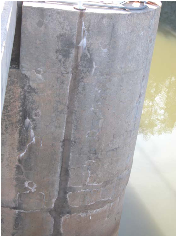
54. Afterbay Dam – East side Pier 2, upstream.
