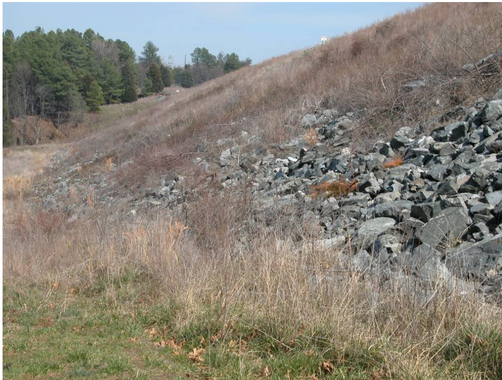
28. West Ash Pond Dam – Downstream slope and toe.
