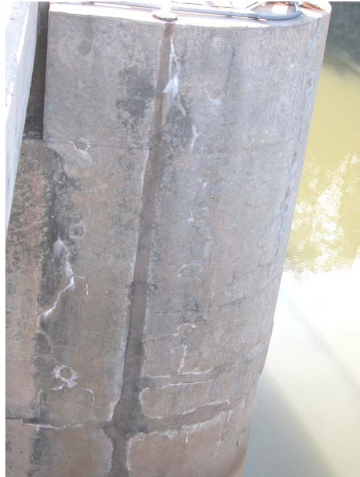
57. Afterbay Dam – West side Pier 3, upstream.
