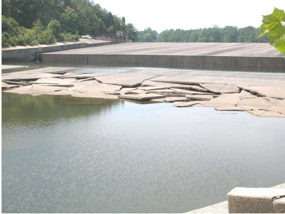
9. Main Dam – Lower spillway (August 5, 2008).
