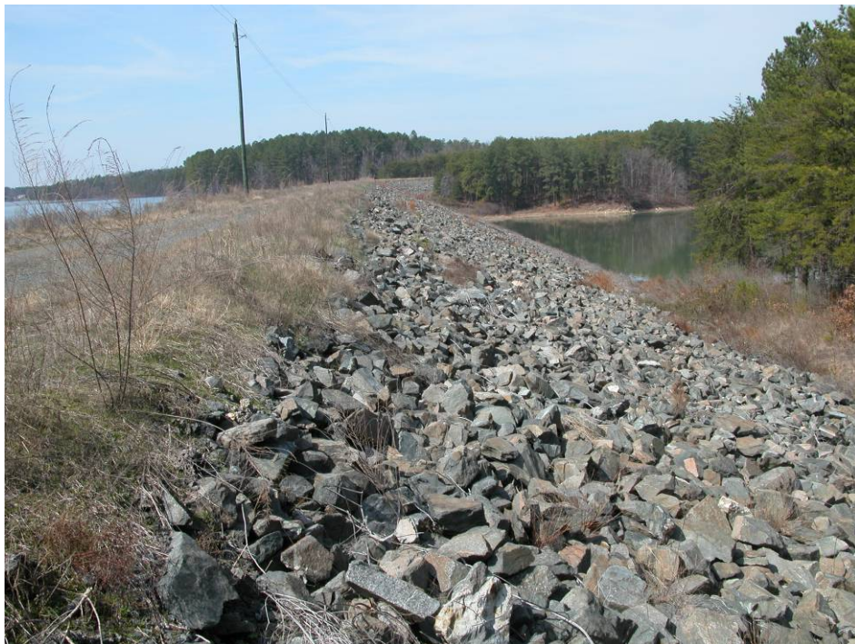
2. Main Dam – Crest and downstream slope looking west.
