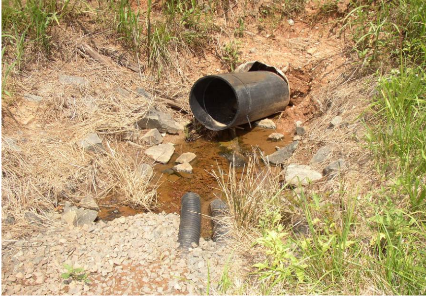
#35 Seepage Collection Area Near Maximum Section of Downstream Toe of East Dike
