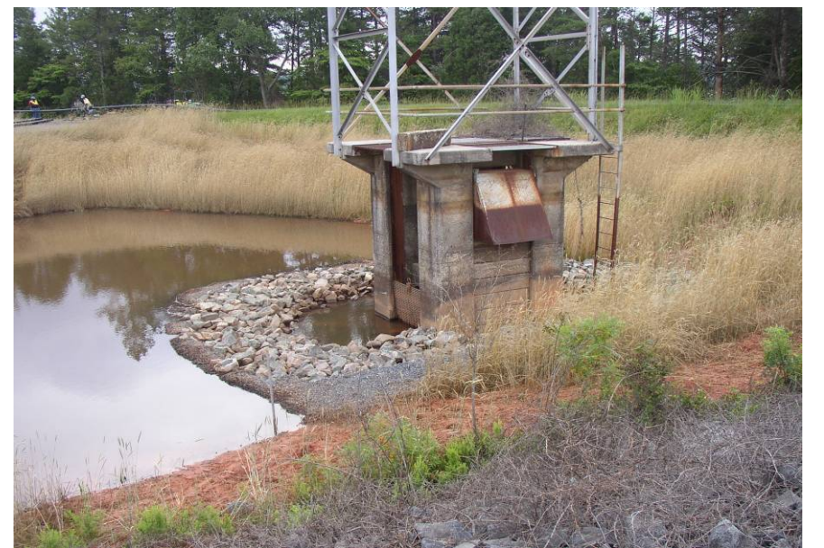
#55 Drop Inlet for Retained Ash Basin
