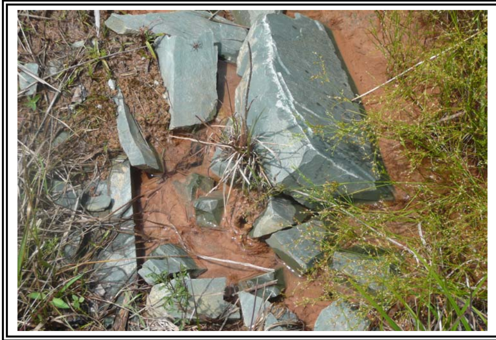
Seepage at the toe of the secondary dike about 300 feet from piezometer row. Water is clear.
