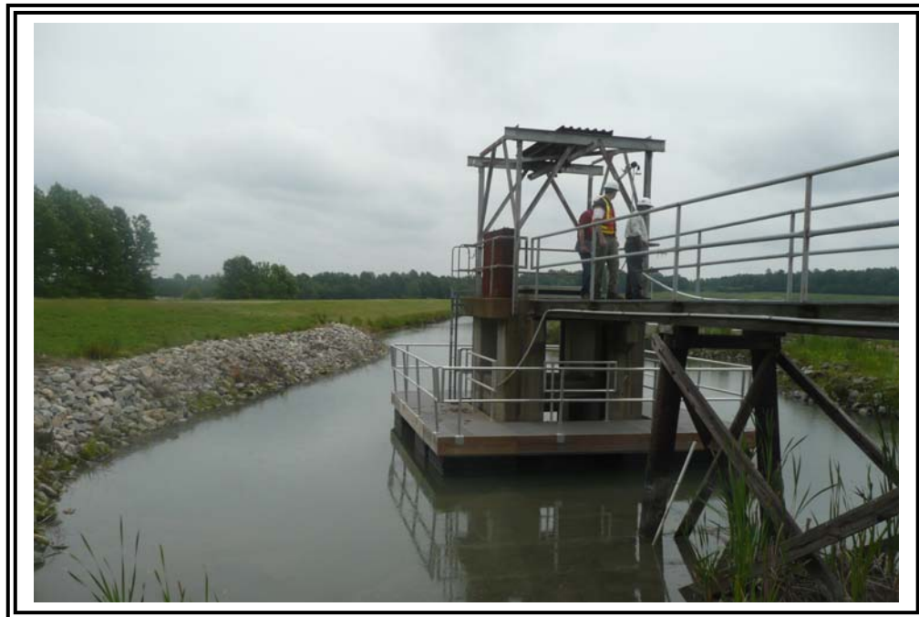
Primary pond outlet tower at north corner of the pond.
