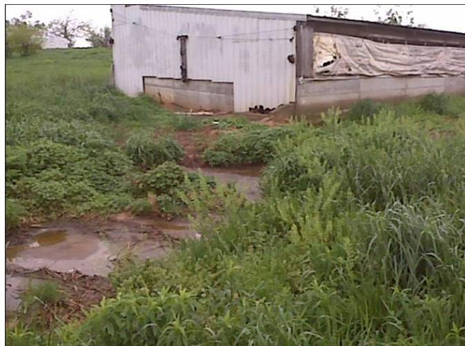
**Photo 8.** An in-house pit in this swine barn is designed to have manure transported from the pit to an earthen storage structure through a pipe. Due to a pipe break, manure is leaking and flowing downhill from the barn. (Source: EPA Region 5.)
