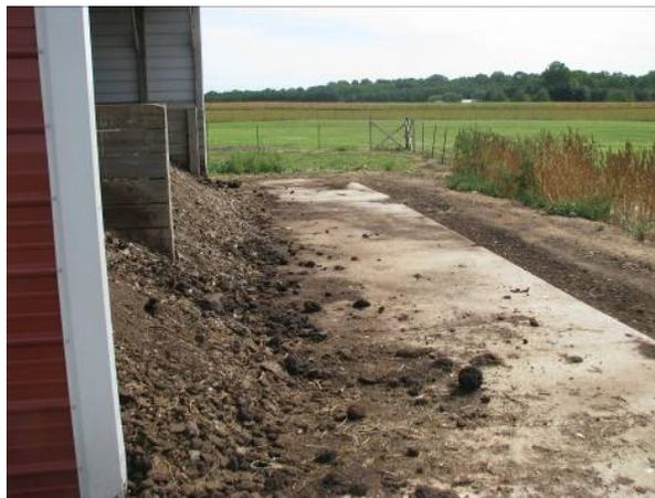
**Photo 9.** This storage structure may have inadequate capacity for the amount of litter being stored. The area around the storage shed drains to a water of the U.S. and does not have any runoff controls. (Source: EPA Region 3.)
