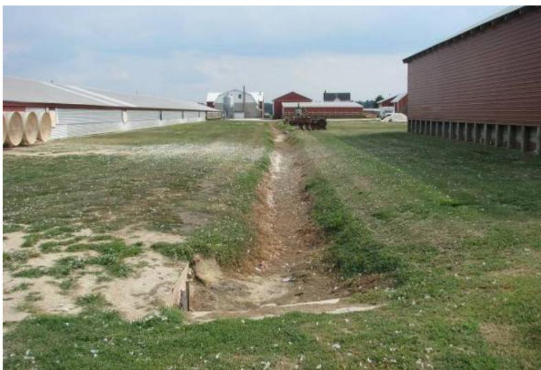
**Photo 10.** The photo shows a poultry operation that was designed to have precipitation drain away from houses through a conveyance system that discharges to a water of the U.S. If pollutants will be carried by this conveyance system to waters of the U.S., the facility is proposing to discharge. (Source: EPA Region 3.)
