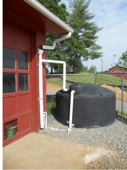
Figure 6. Rain Barrel and Cistern Setup
