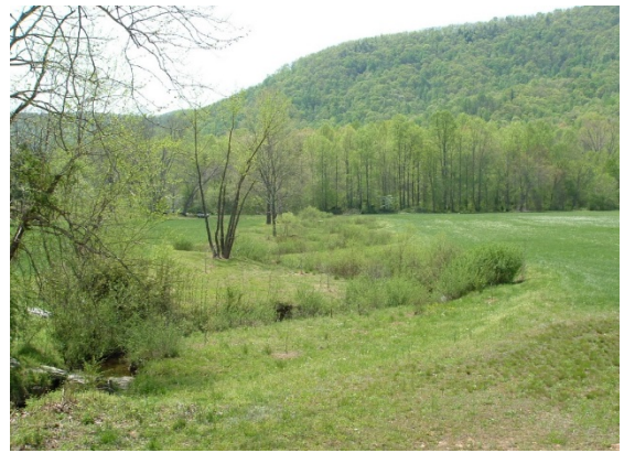
Meandering Vegetated Channel Three Years After Restoration
