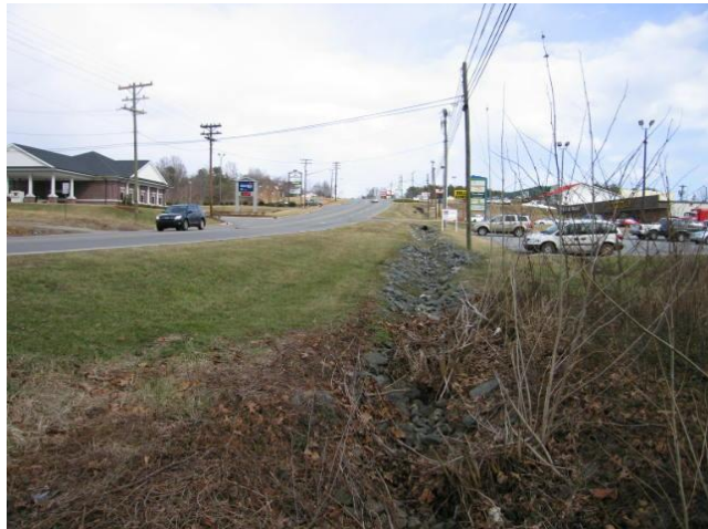
Photo 3. Rock lined stormwater ditch along NC 268 that discharges directly to Heatherly Creek at NC 268.
