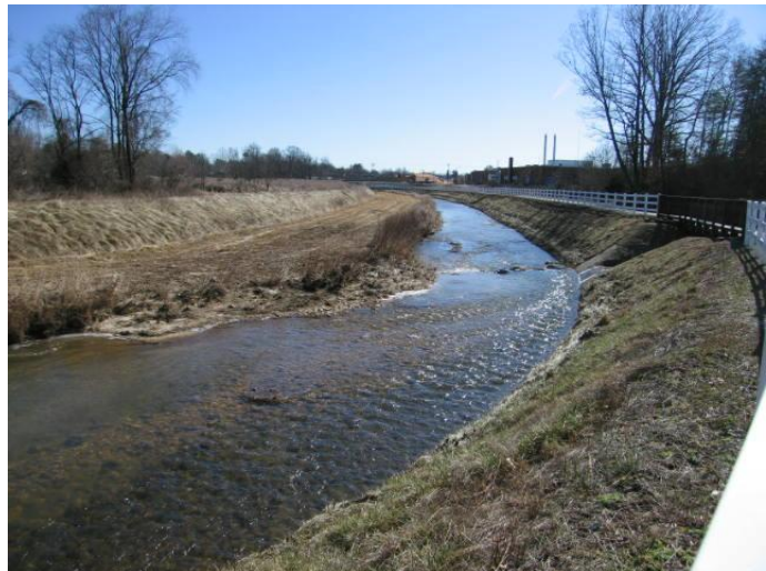
Photo 6. Lovills Creek in an engineered flood control channel.
