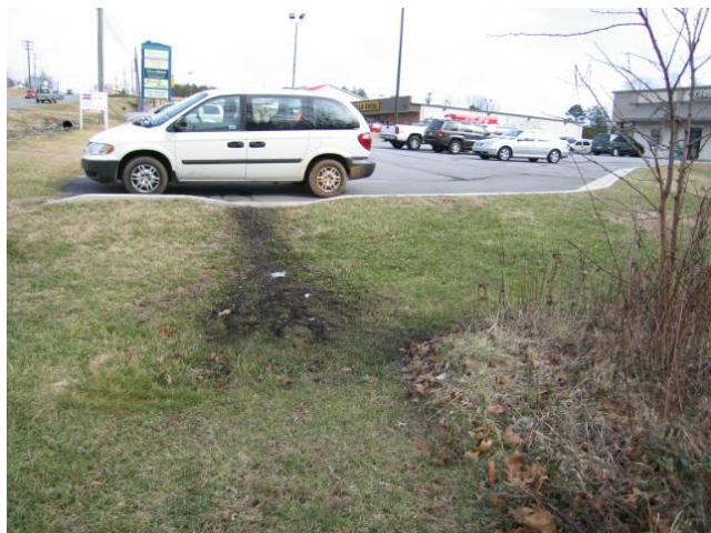
Photo 4. A grass filter strip (providing some unintentional filtration) that may be suitable for retrofitting to provide improved treatment of runoff from the parking lot.
