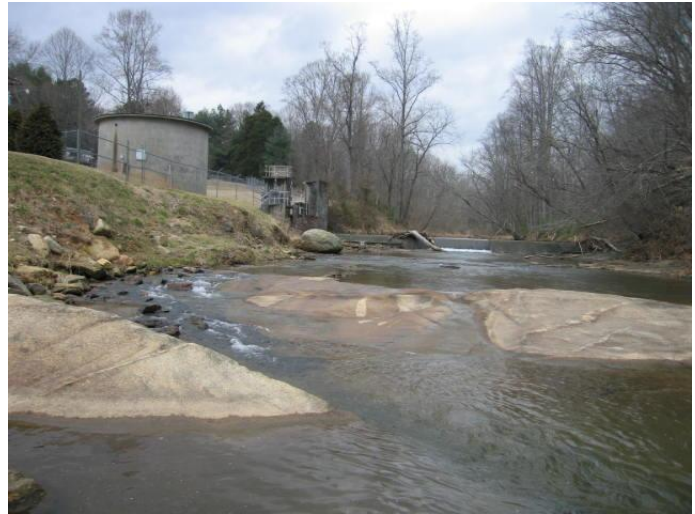
Photo 9. Mount Airy pump station and low flow dam at upstream end of engineered channel in Lovills Creek.
