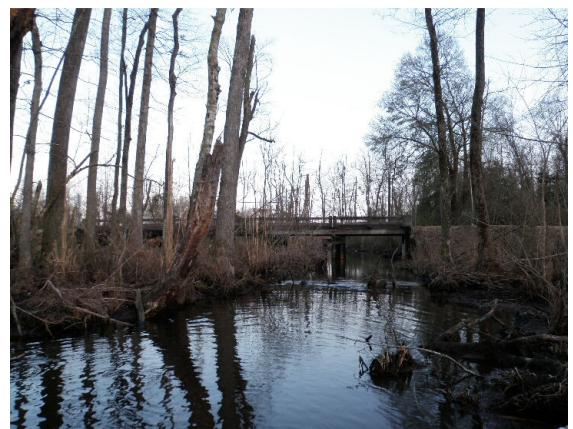
Figure 4. Great Coharie Creek at SR 1703 (GCC1703) looking downstream.
