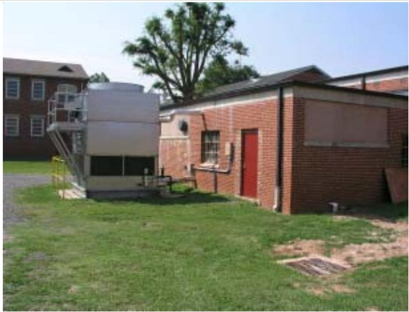
Pipes leading from kitchen to cooling tower and pump station. (Dirt path shows where excavation took place for laying the pipes.)
