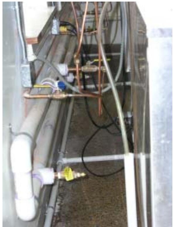
Pipes behind centralized ice machines, connecting cooling loops.
