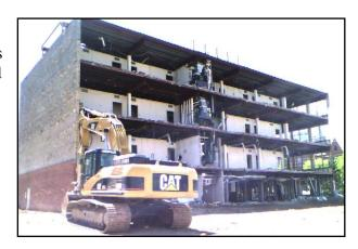
The development of this site required the removal of two existing buildings located in the development footprint. With the goal of recycling as much of the construction and demolition waste as possible, a construction and demolition materials management plan was put into place, and adopted as part of the contracting documents.
