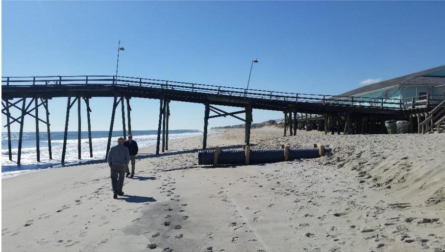
Fig. 2 Exposed outfall pipe and framing on an eroded beach
