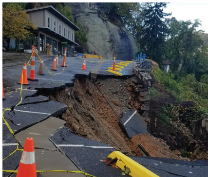
Landslide damage to Chimney Rock parking lot
