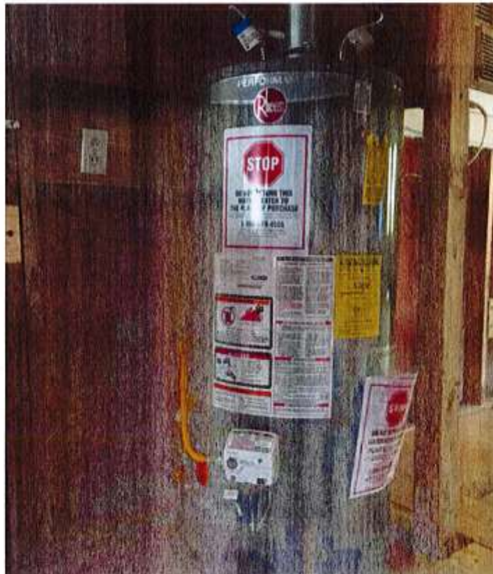
Example Water Heater Replacement under STEP in Unfinished Area
